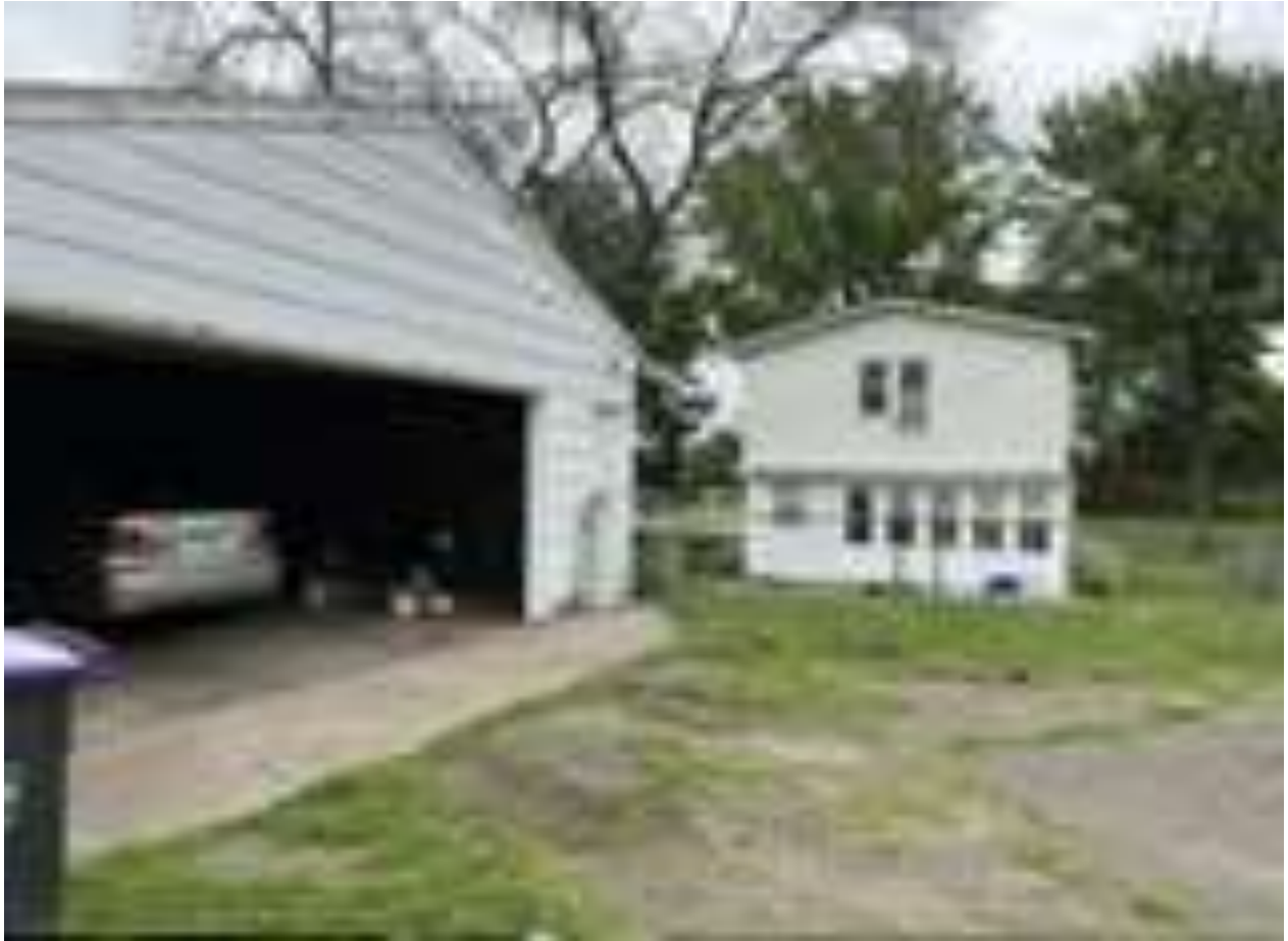
1872 Clear Ave photos 7-22-25
