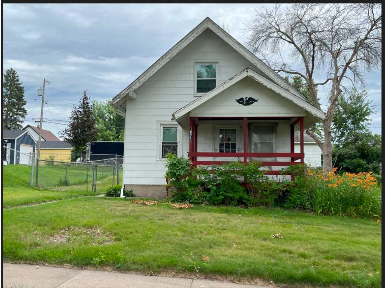
1872 Clear Ave photos 7-22-25
