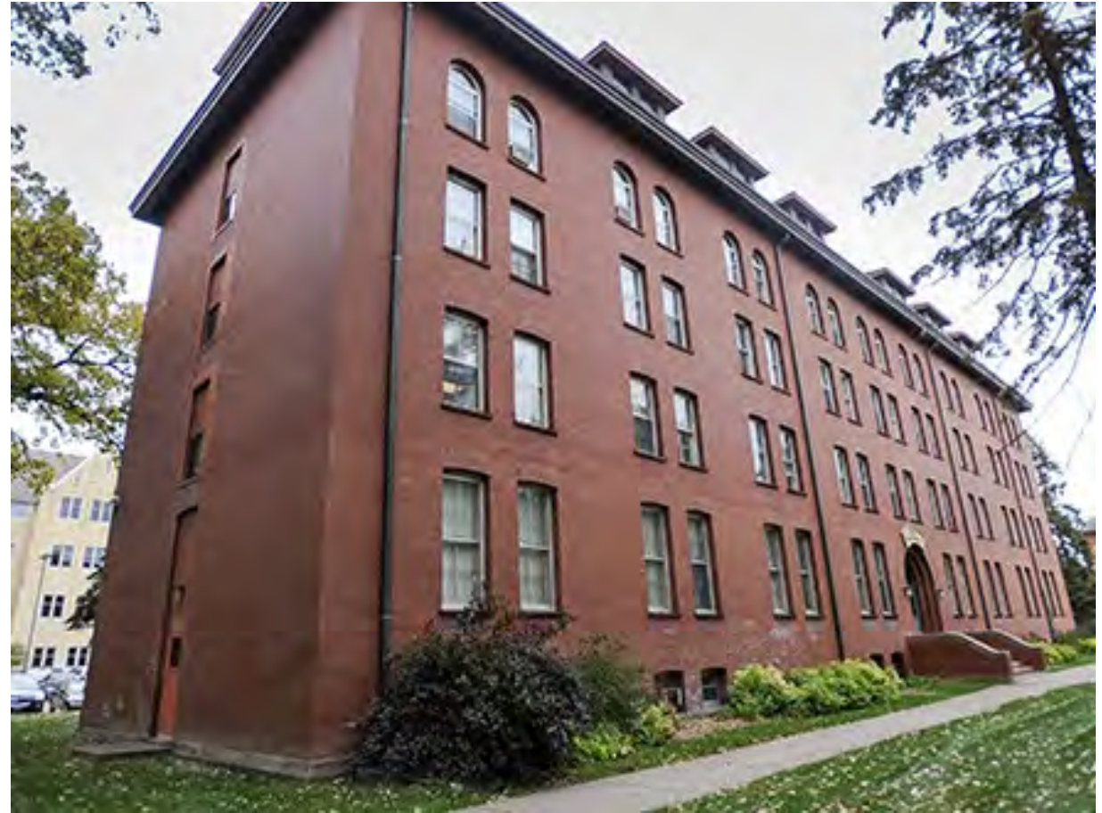
View from NW corner
