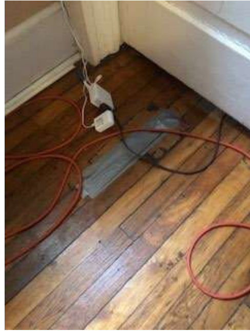
33: Tape to repair flooring in tenant unit
