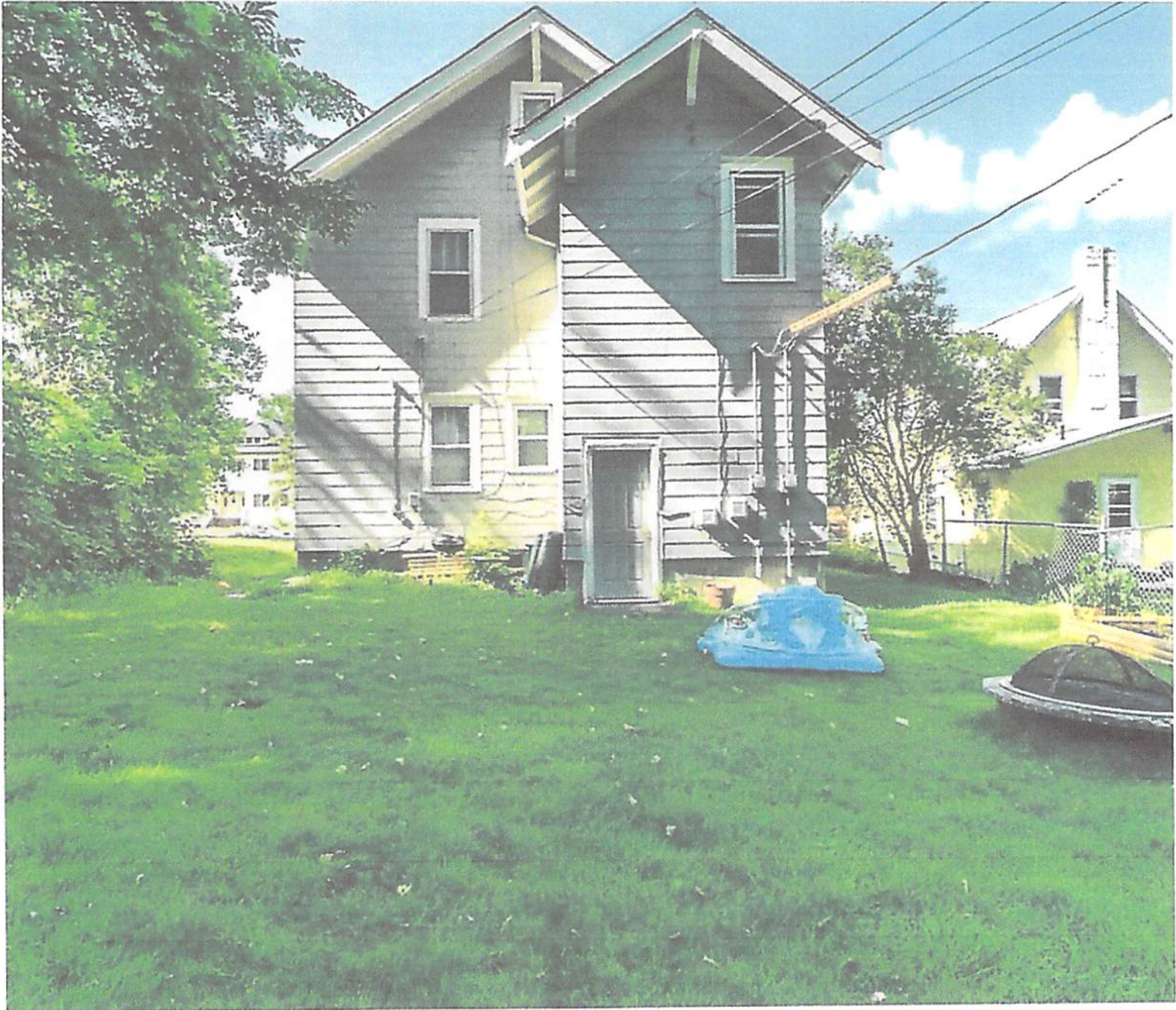
Backyard from garage point of view.
