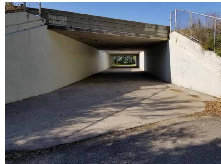
Segment 1/2 : MnDOT owned trail underpass below Hwy 61
