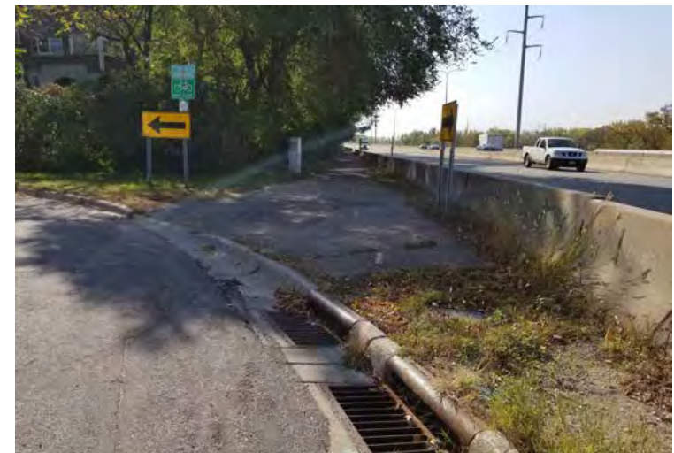
Segment 3B narrow right of way between Hwy 61 & Pt Douglas.
