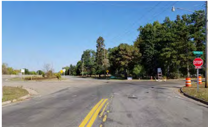
Point Douglas Rd at Carver Avenue
