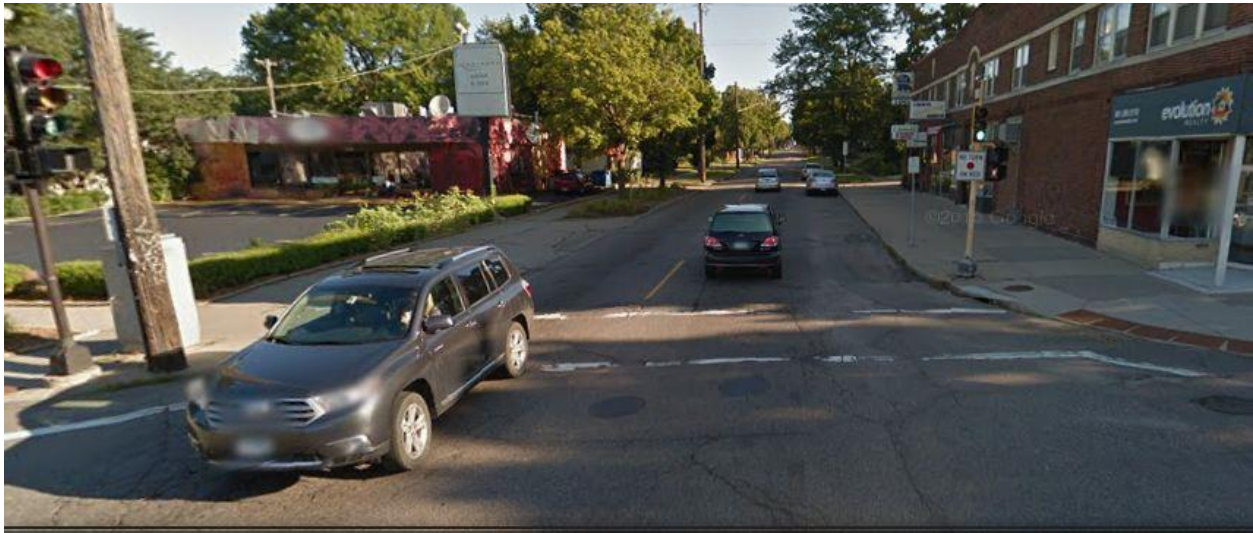
Photo credit: Google Maps . Southbound cars cannot drive around a turning vehicle stopped too close to the crosswalk.
