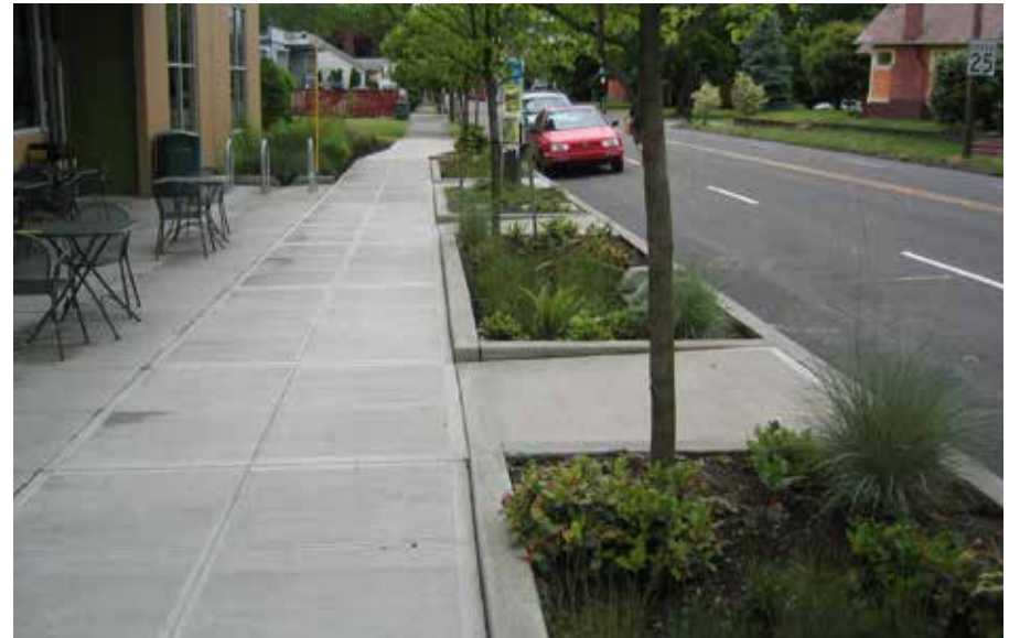
Examples of infiltration and flow-through planters
