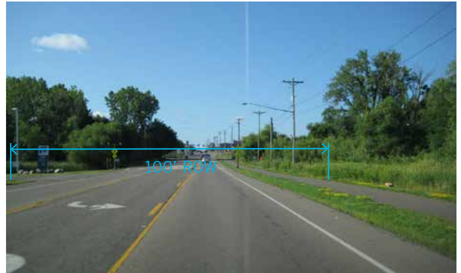
Photo of existing Rice Street 100' ROW (north of Larpenteur Avenue)
