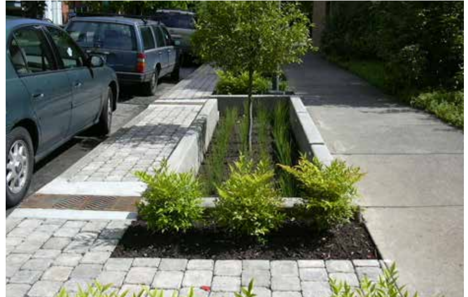
Examples of infiltration and flow-through planters
