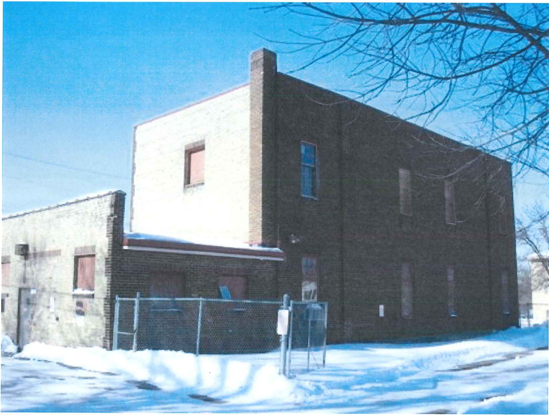
Subject site from alley, facing northwest
