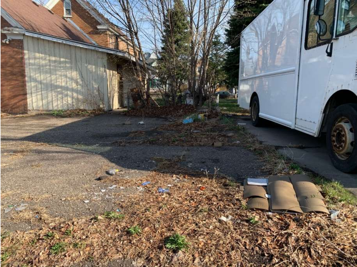
678 Lafond Ave.Rechecked Photos.4-6-21
