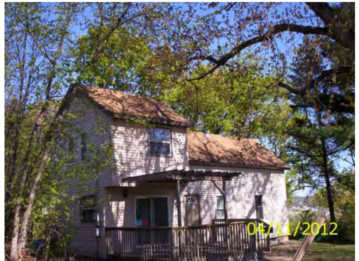
South and east sides, posting
