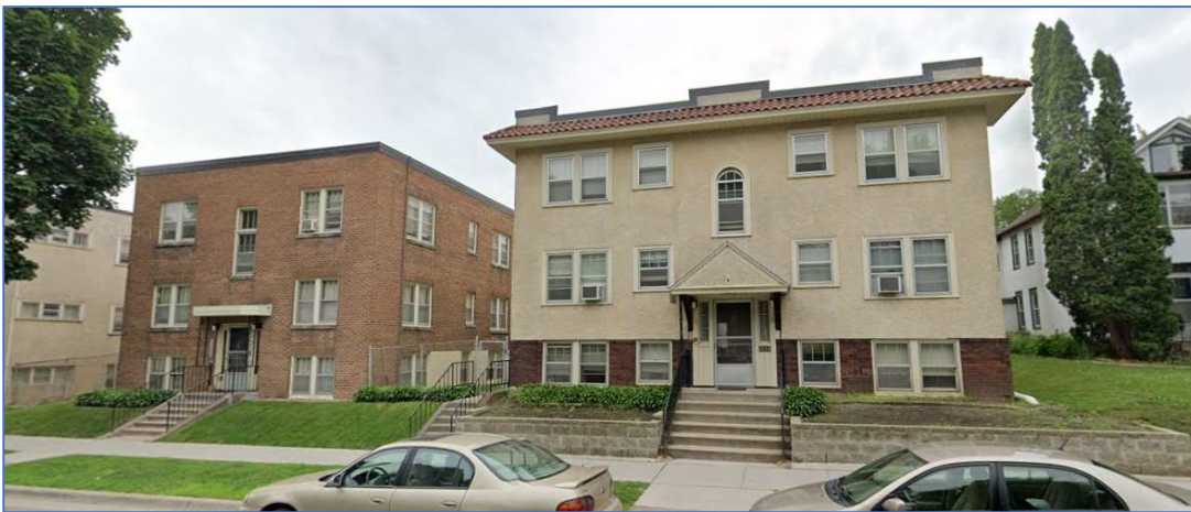
1848 St. Clair Ave – 14 units built in 1938 (~5' side yard on west side) & 1854 St. Clair Ave – 10 units built in 1935 (~4' on east side and ~5' on west side)
