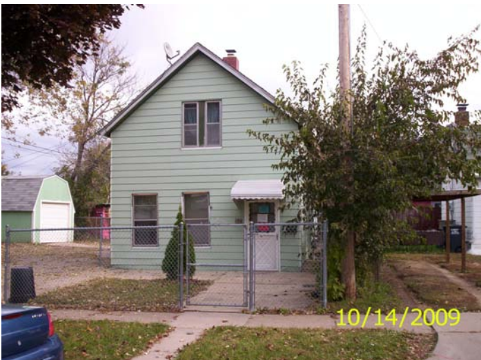
West and south sides, postings
