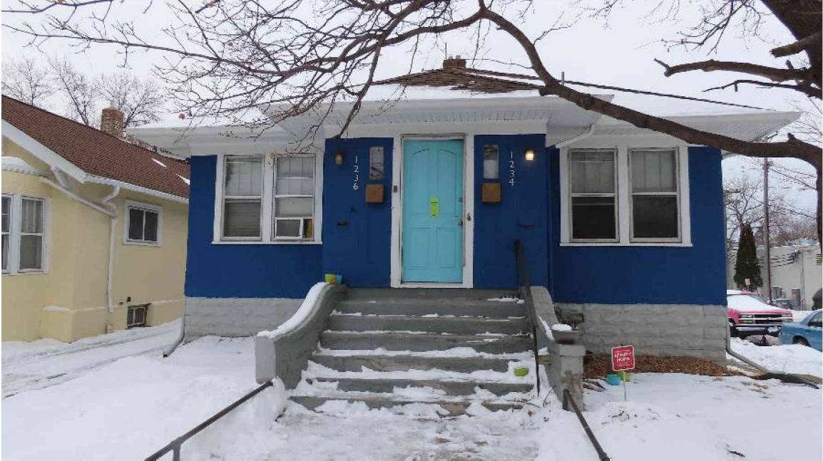
Photograph 1: Front, west-facing side of the house.
