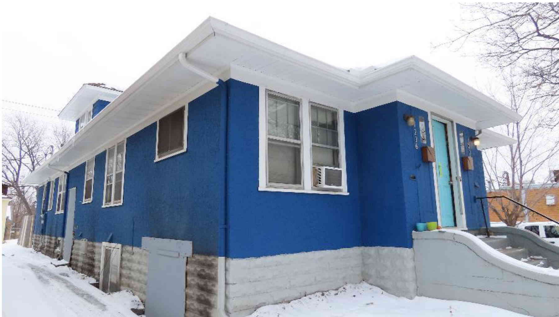
Photograph 4: North and west sides of the house.
