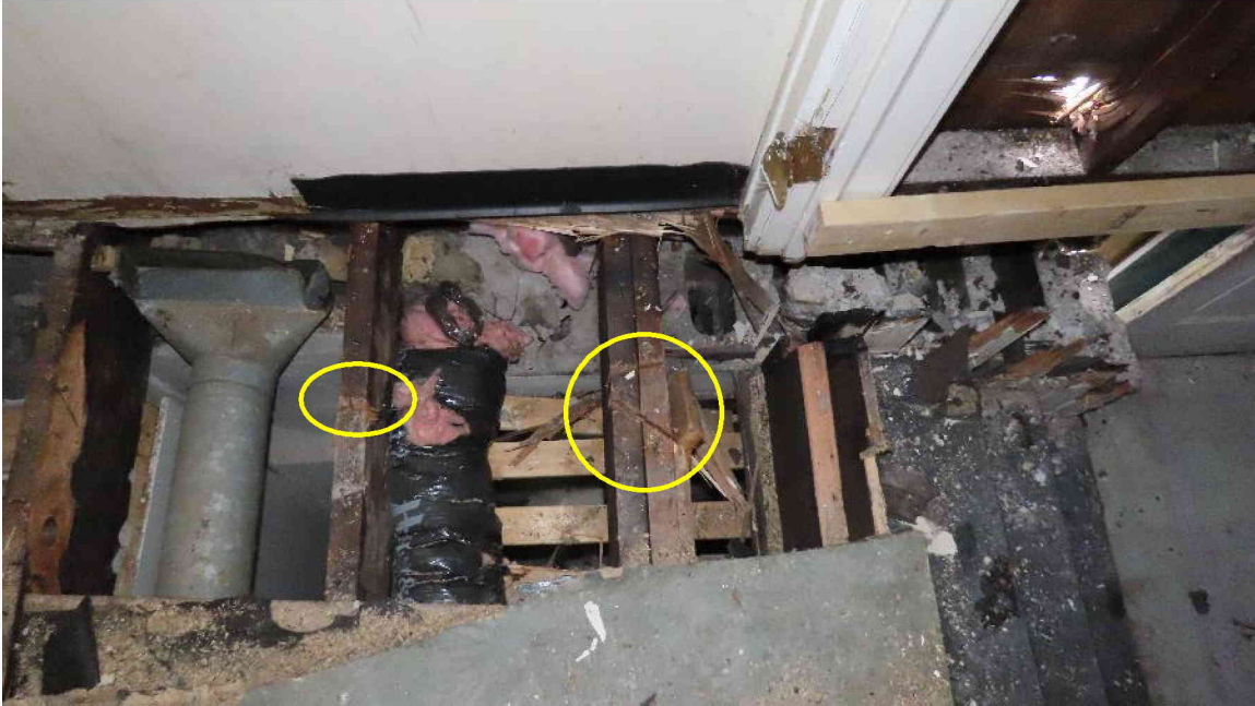
Photograph 13: Sawcut in floor joists.
