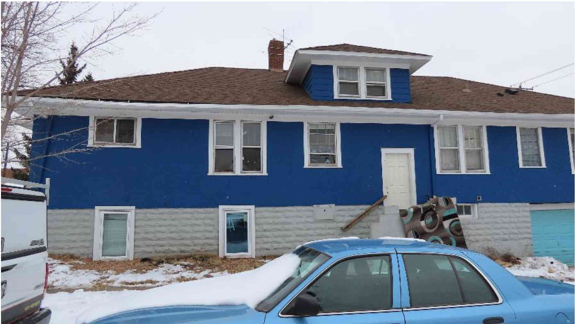
Photograph 2: South side of the house.
