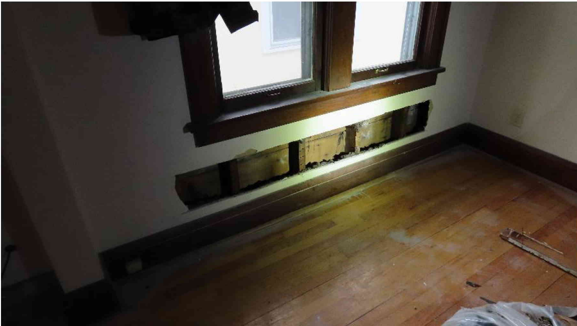
Photograph 10: Drywall removed from the north wall under the dining room window.
