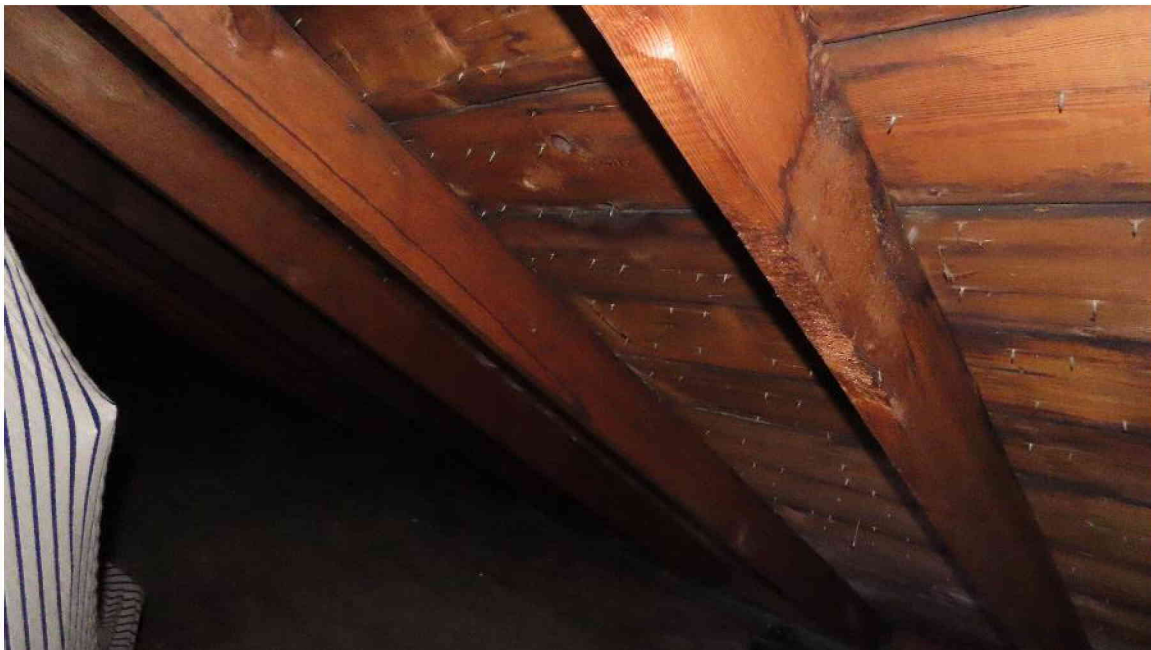
Photograph 18: Exposed north roof slope rafters in the attic.
