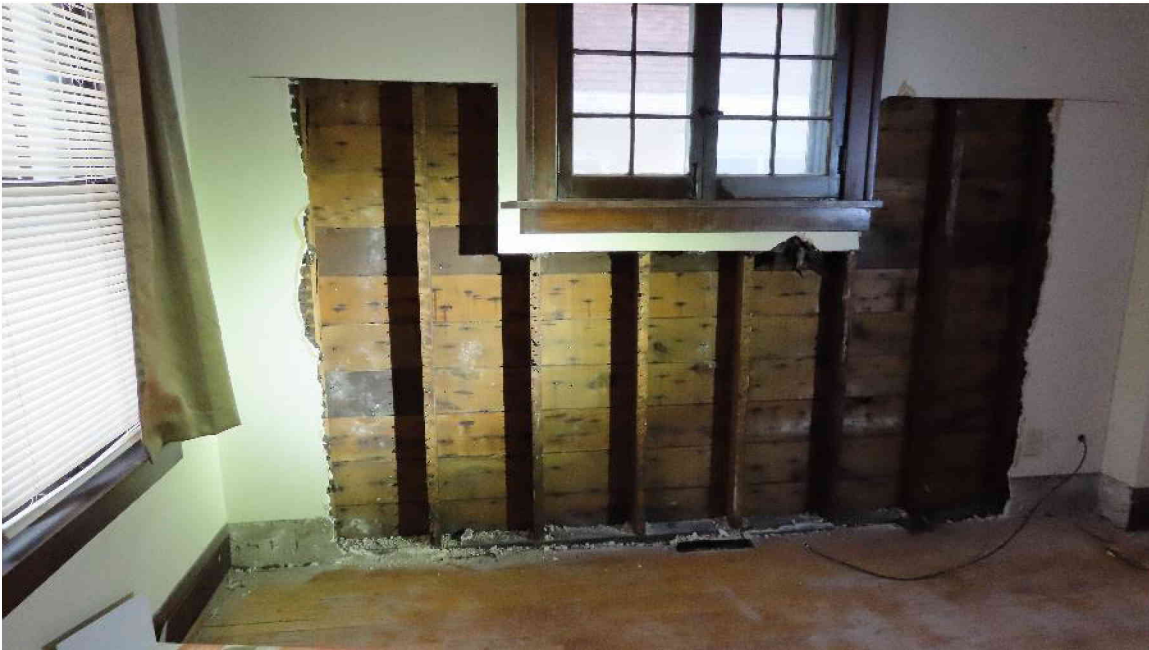
Photograph 8: Drywall removed from the north wall of the living room.
