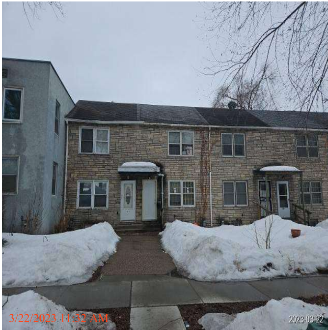
Address: 1008 CARROLL AVE SAINT PAUL MN 55104 Date Completed: 03/22/2023 Description: FRONT OF HOUSE front of house
