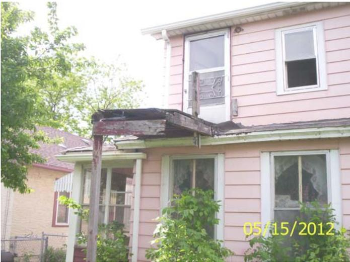
**Deteriorated and missing 2<sup>nd</sup> floor porch/steps/rails**
