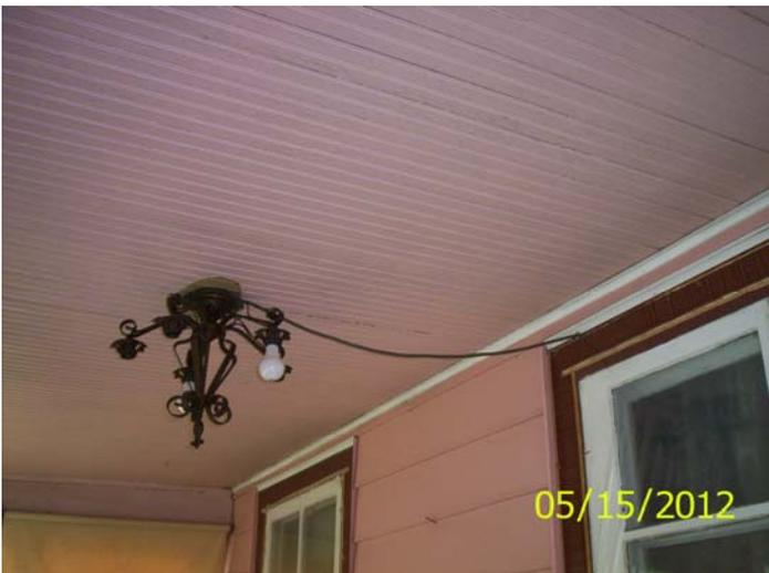
**Extension cord wiring to light fixture**
