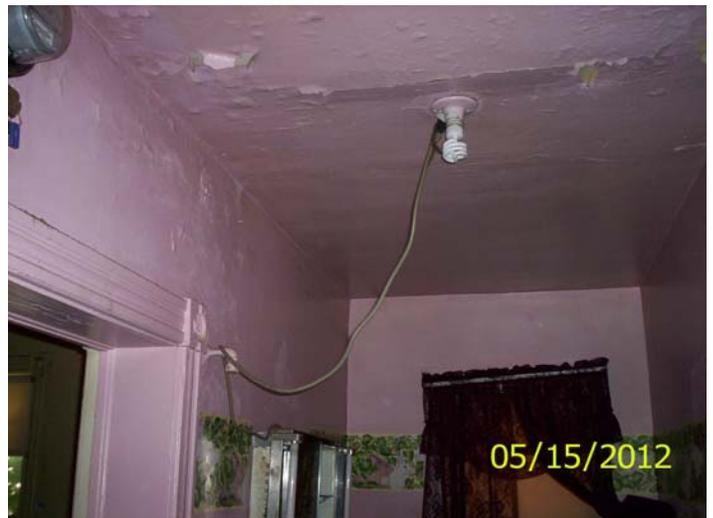
Extension cord wiring to light fixture
