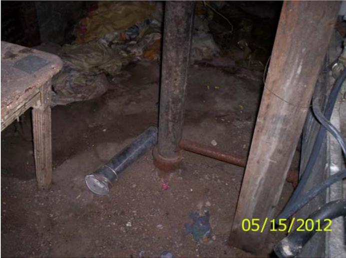
**Water on dirt floor, improper drain into stack**
