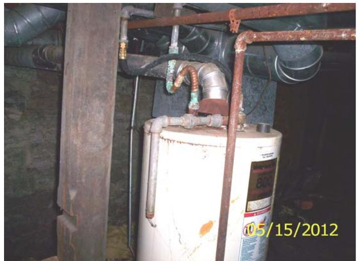
**Improper water heater installation**
