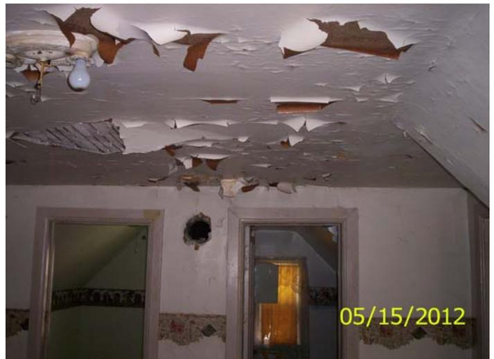
**Water damaged ceiling, open chimney**
