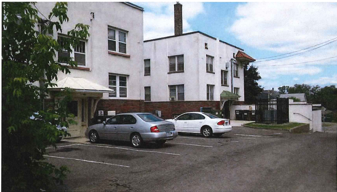
Multifamily buildings to the east of the subject property (rear)
