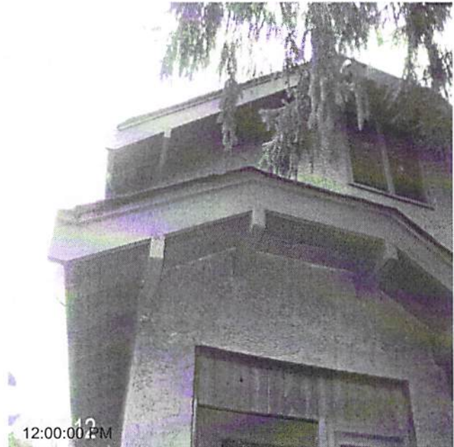
Date Completed: befroe: prep&paint exterior trim
