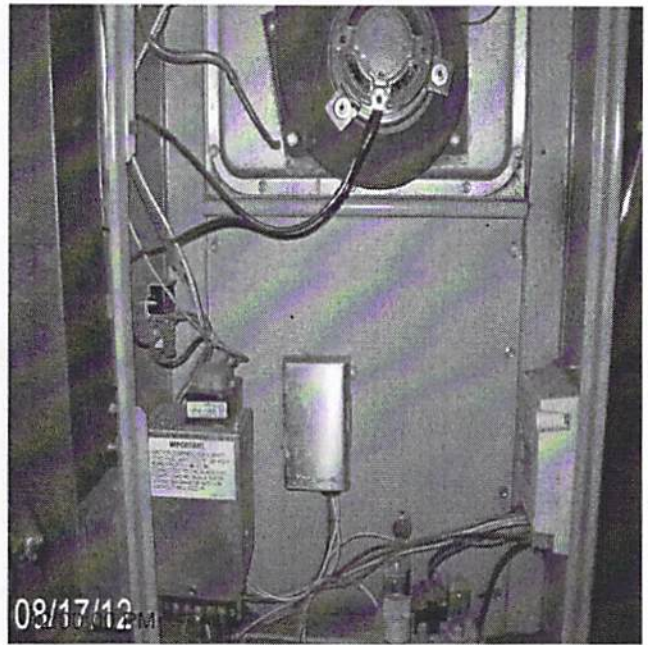
Date Completed: before install furnace filter
