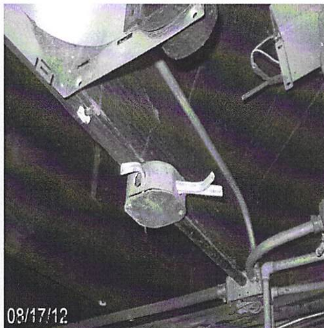
Date Completed: before: rewire
