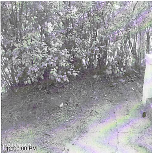
Date Completed: before: grade landscape
