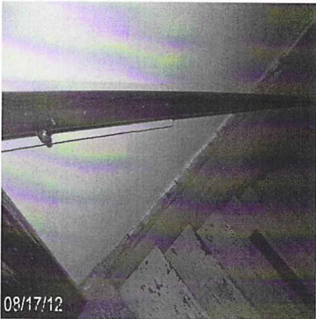
Date Completed: before: install handrail in entryway
