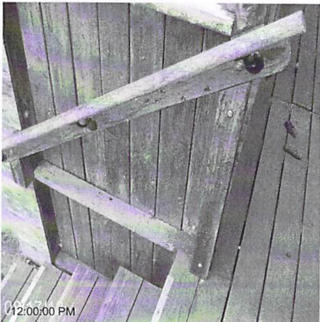
Date Completed: before: install handrail in entryway
