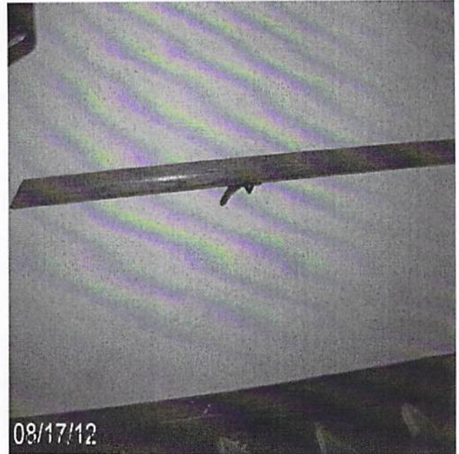
Date Completed: before: install handrail in entryway
