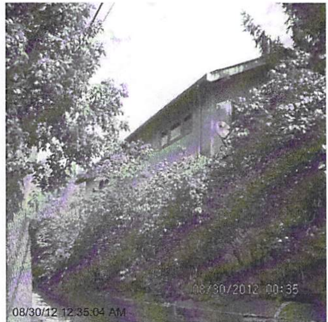
Date Completed: 09/03/2012 side of home
