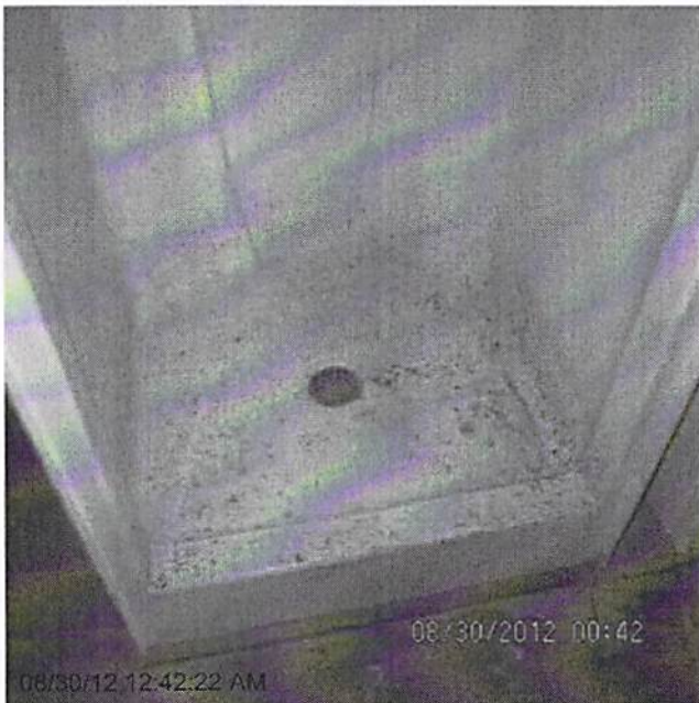
Date Completed: 09/03/2012 mold-bleach and kilz 624 sq ft of mold using 2 gal
