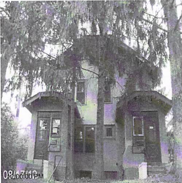
Date Completed: before: prep&paint exterior walls
