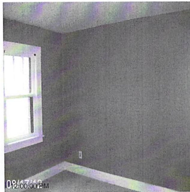
Date Completed: before: prep&paint walls upstairs
