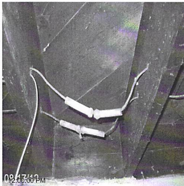
Date Completed: before: rewire
