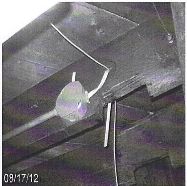
Date Completed: before: rewire
