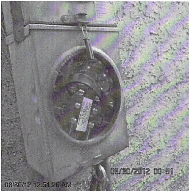
Date Completed: 09/03/2012 missing elec meter
