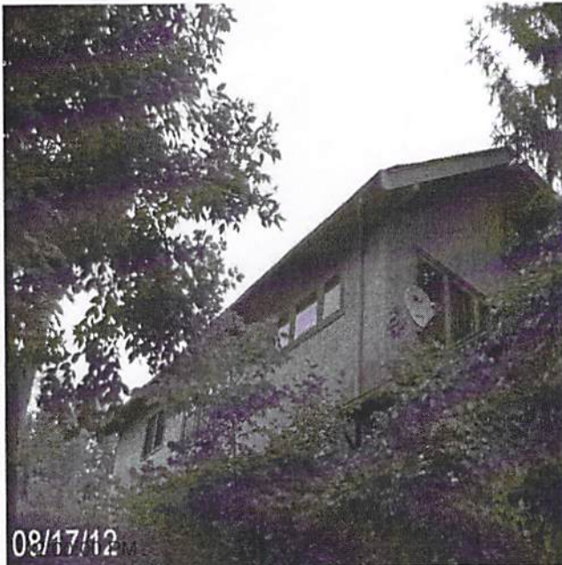
Date Completed: before: install down spouts
