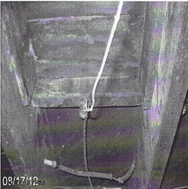
Date Completed: before: rewire
