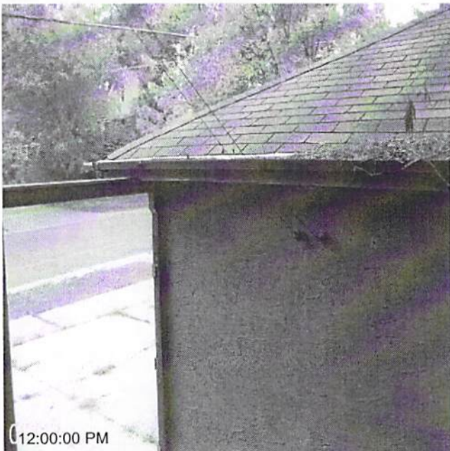
Date Completed: before: install garage circuit
