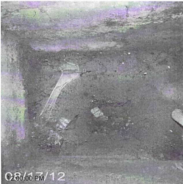
Date Completed: before: cover water pit with concrete
