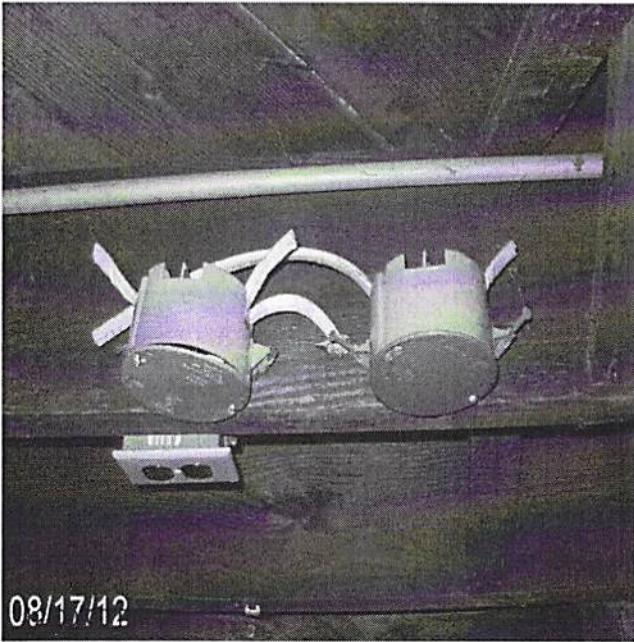
Date Completed: before: rewire
