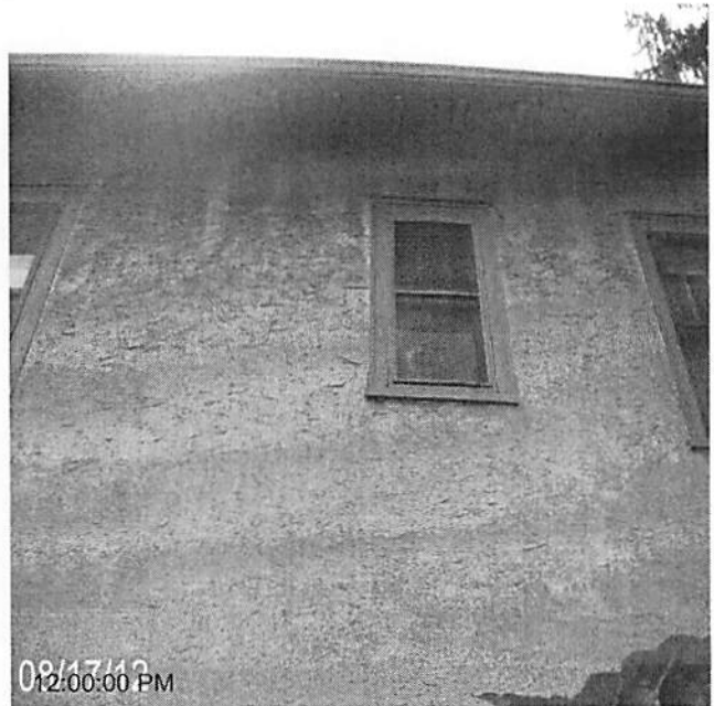
Date Completed: before: replace window screens upstairs
