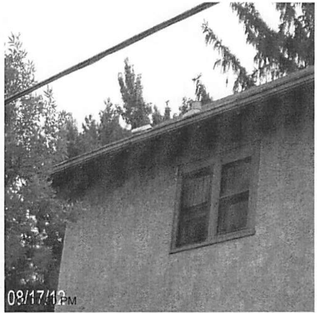
Date Completed: before: install gutters
