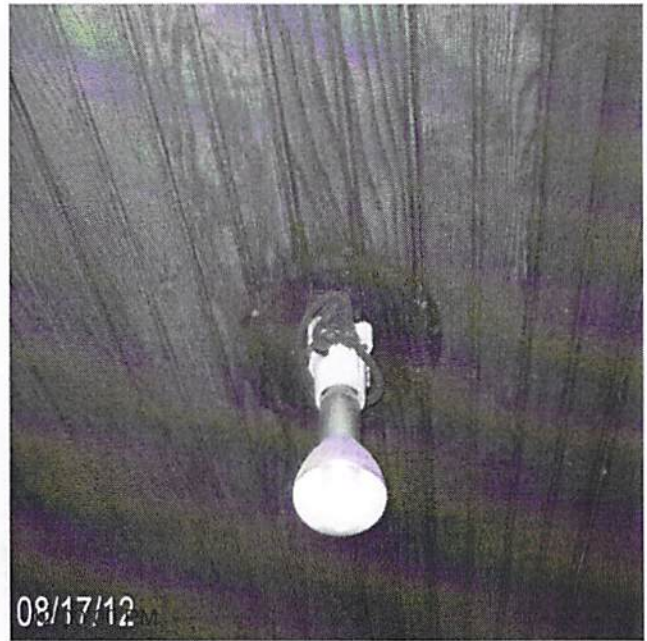
Date Completed: before:rewire to standard attic
