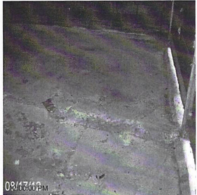
Date Completed: before: level garage floor
