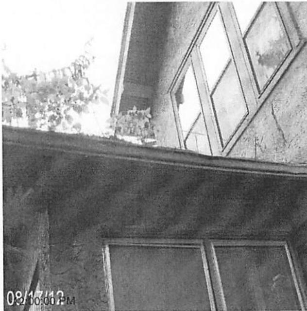
Date Completed: before: install gutters
