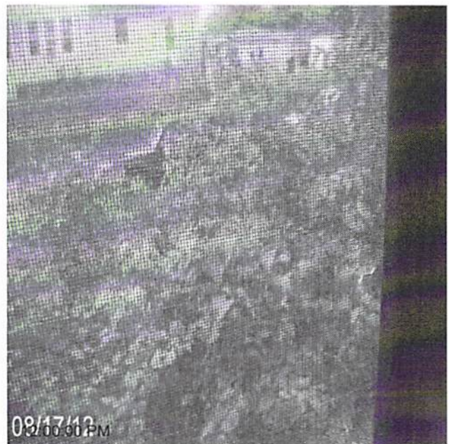
Date Completed: before replace window screens upstairs
