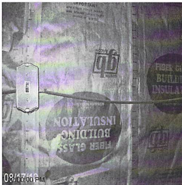
Date Completed: before:
