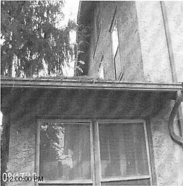
Date Completed: before: install gutters
