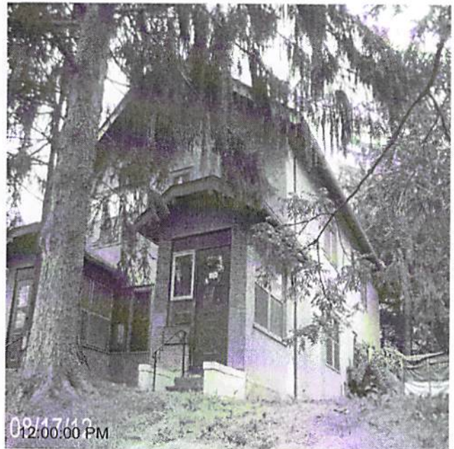
Date Completed: before: prep&paint exterior walls
