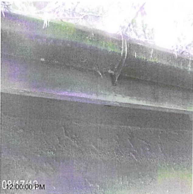
Date Completed: before: prep&paint exterior trims
