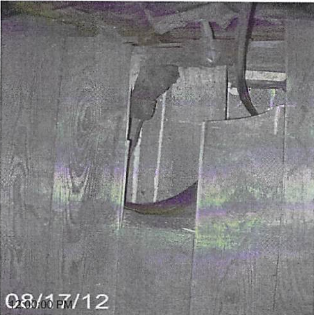
Date Completed: before: insulate attic floor
