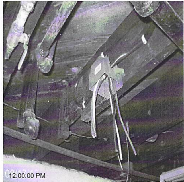
Date Completed: before: rewire
