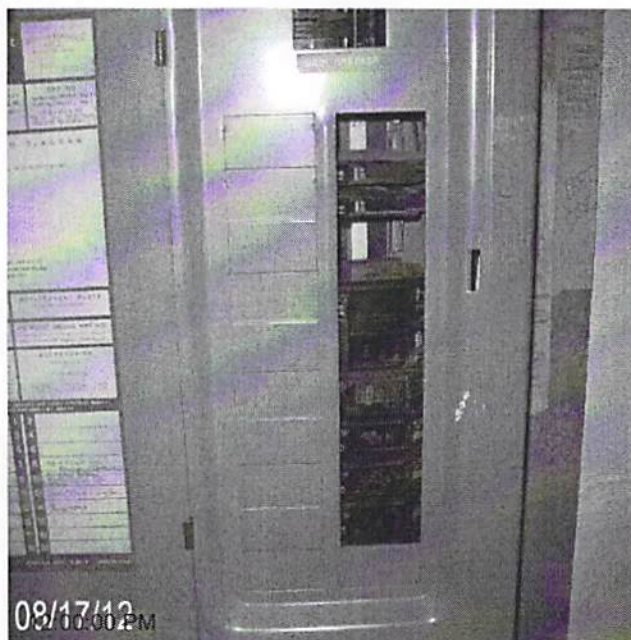
Date Completed: before: circuit breaker amp
