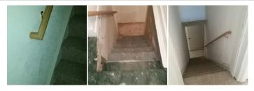
I5. There Are Missing Or Defective Guardrails. Provide All Stairways, Porches, Decks Or Steps Which Are More Than 30" High With Guardrails And Intermediate Rails With Openings In The Guardrail No More Than Four (4) Inches Apart And In Accordance With The State Building Code. Total: \$383.32
