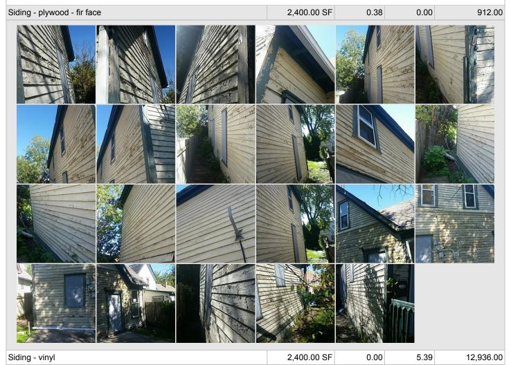
E6.The Exterior Walls Of The House And/Or Garage Are Defective. Repair All Holes, Breaks, Lose Or Rotting Siding, To A
