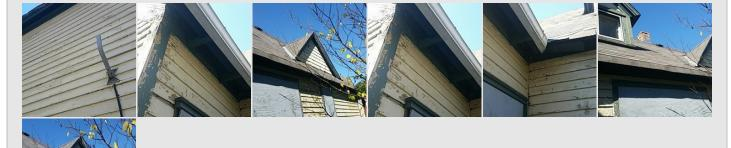
E2.The Eaves And Soffits Are In A State Of Disrepair Or Deterioration. Repair All Defects, Holes, Breaks, Loose Or Rotting Boards, To A Professional State Of Maintenance. Permit May Be Required. Total: \$2,219.50
