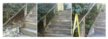
I6. The Stairs Have Missing Or Defective Handrails. Provide All Interior And Exterior Stairways And Steps Of More Than Three (3) Risers With Handrails Which Are Grippable And Installed 34" To 38" Above The Nose Of The Stair Treads. Total: \$616.64
