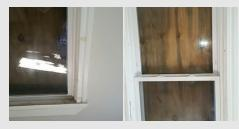
E7.The Window And/Or Door Screens Are Missing, Defective Or In A State Of Disrepair. Provide Proper Window And Door Screens For All Openable Windows And Doors. Screens Must Be Tight-Fitting And Securely Fastened To The Frames. Total: \$83.27
