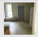
I1.The Bathroom Floor Covering Is Deteriorated Or Inadequate. Provide Floor Covering Which Is Impervious To Water And Easily Cleanable Throughout The Bathroom And Seal Around The Edges And Fixtures. Total: \$4,981.34
