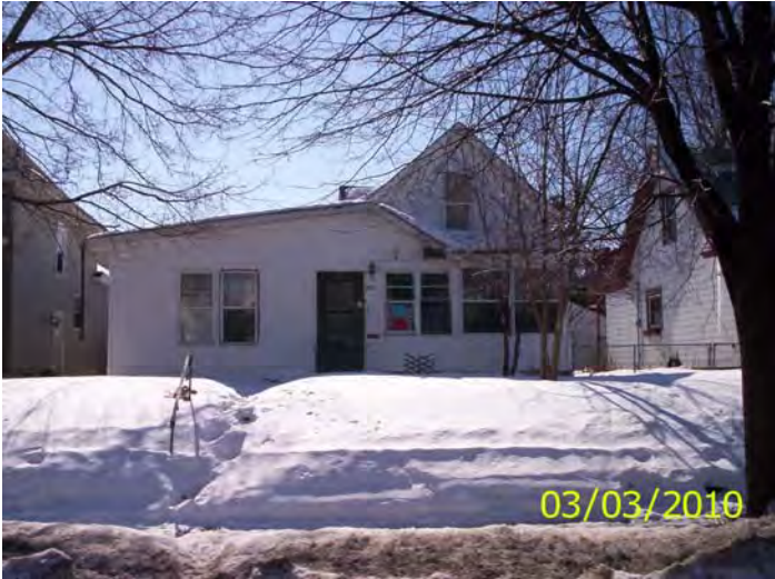
North side, posting
