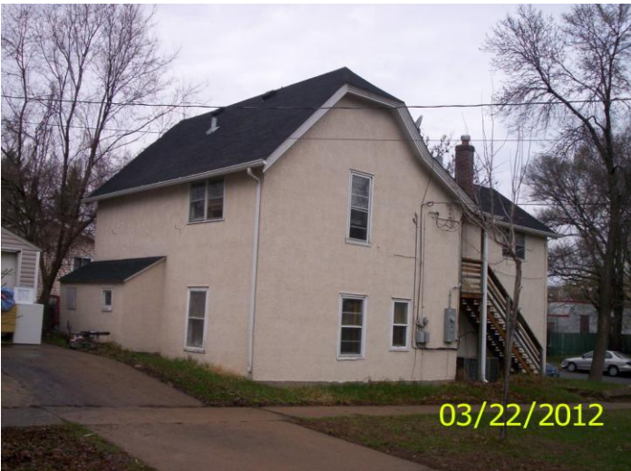
South wall of house
