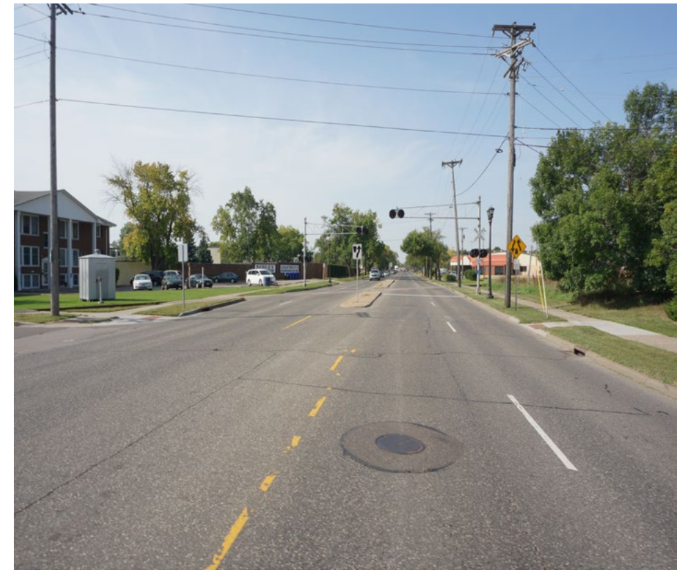
Existing conditions at W 7th Street
