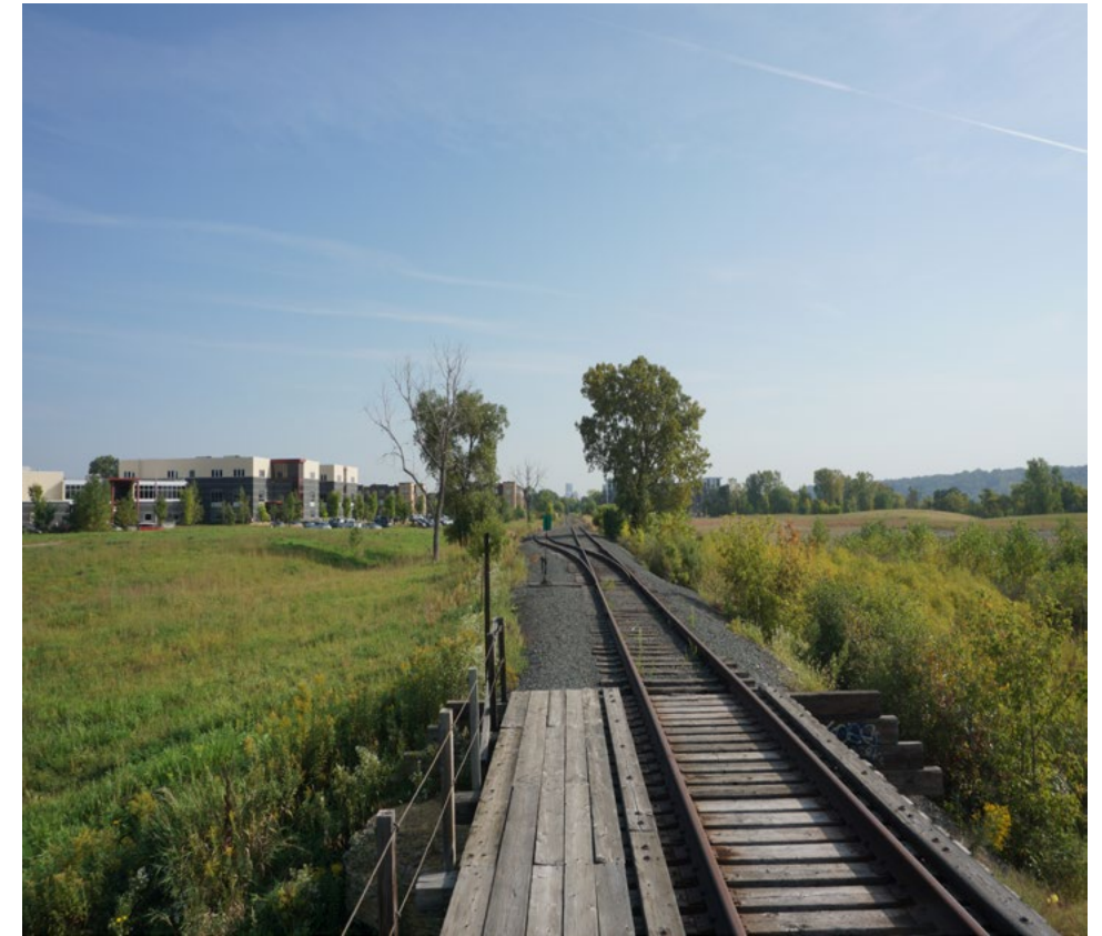
Existing conditions looking northeast towards Victoria Park.
