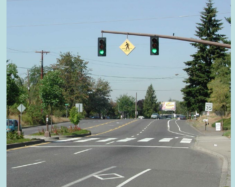
The Springwater Corridor in Portland, Oregon includes high visibility crosswalk markings, pedestrian warning signs, and pedestrian activated signals at crossings.
