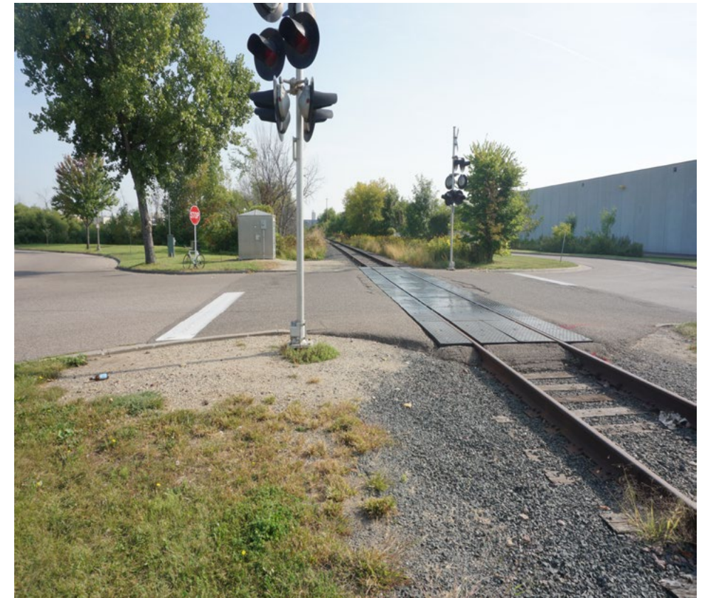
Existing conditions looking northeast at Montreal Way.
