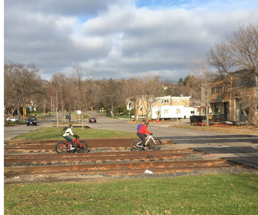
At grade crossing at Edgcumbe may need more formalized infrastructure such as a flashing beacon or pedestrian activated signal.
