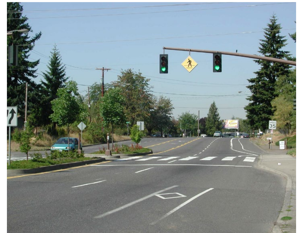
Example of signalized crossing
