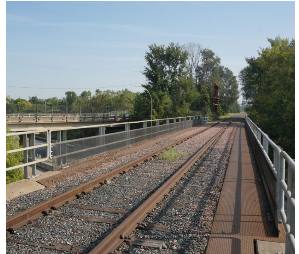
Existing rail bridge over I-35E looking northeast.
