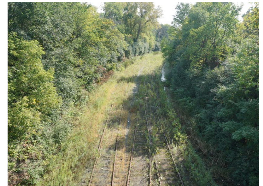
Existing conditions at Cleveland Avenue, looking east
