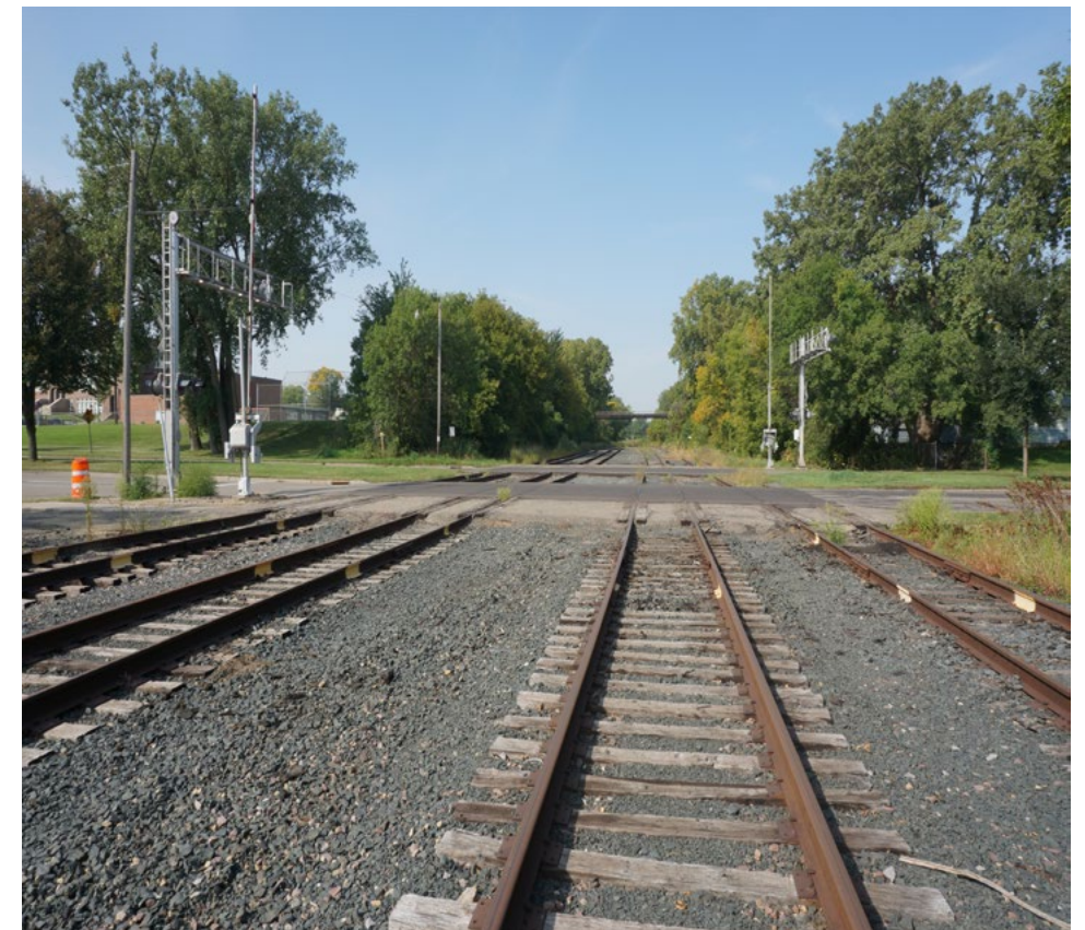
Existing conditions at Edgcumbe Road
