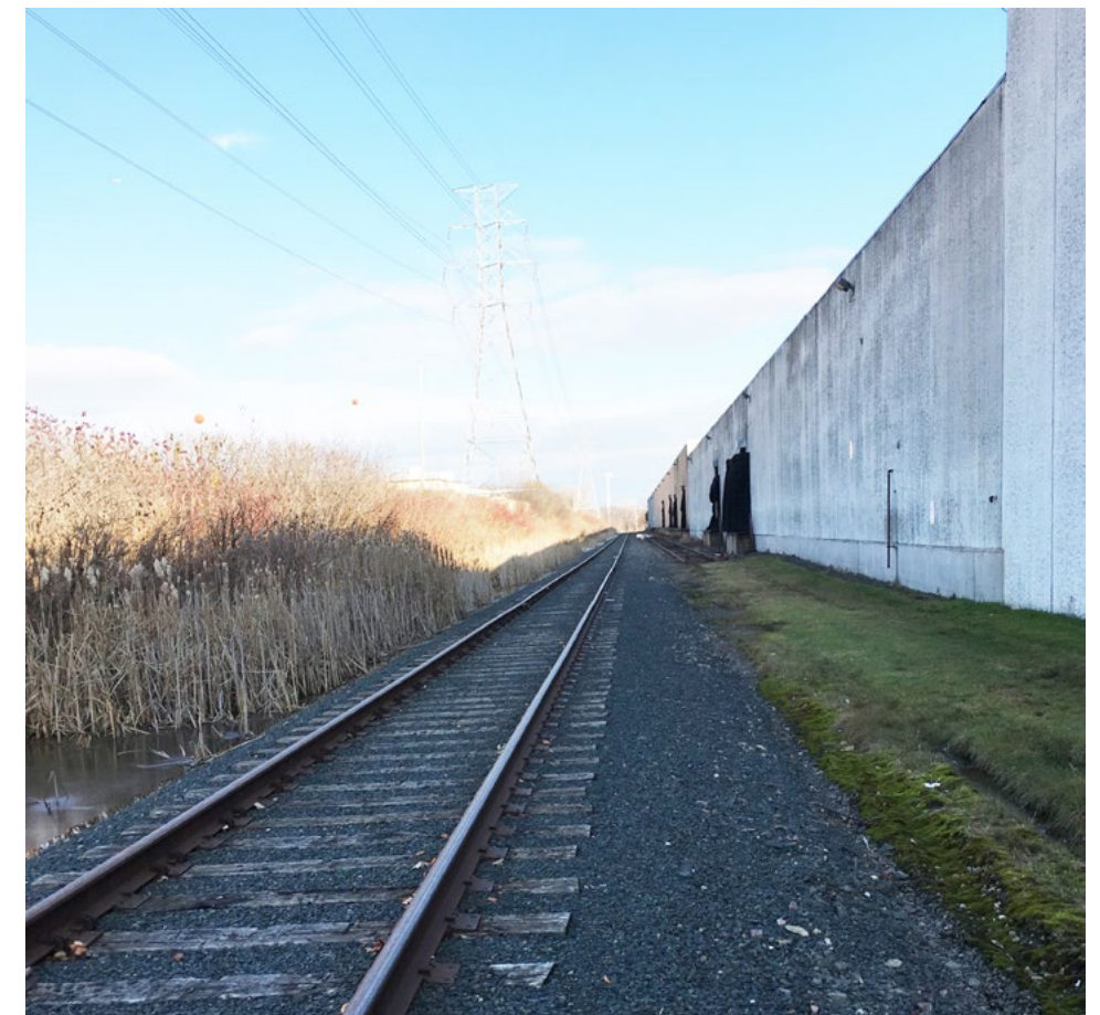
Existing conditions between Rankin and Homer Streets
