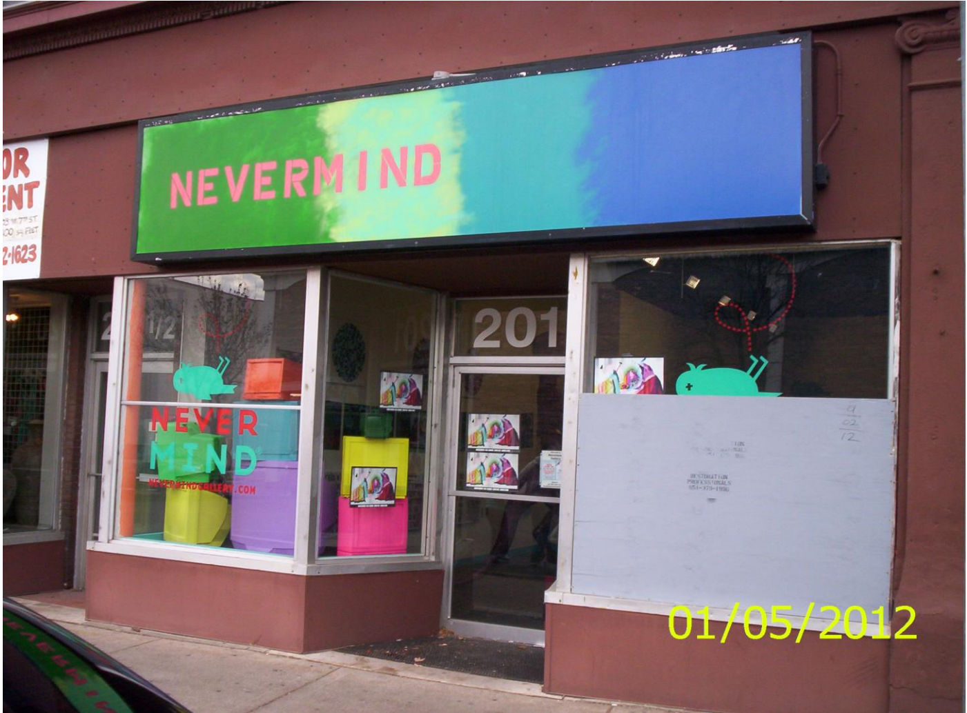
Front of bldg secured
