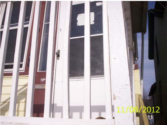
Storm door secured
