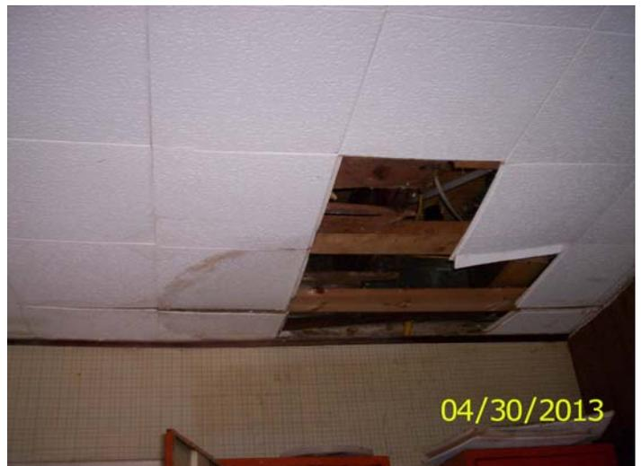
Water damaged ceiling
