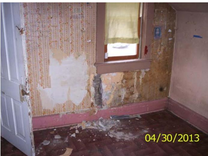
Water damaged wall
