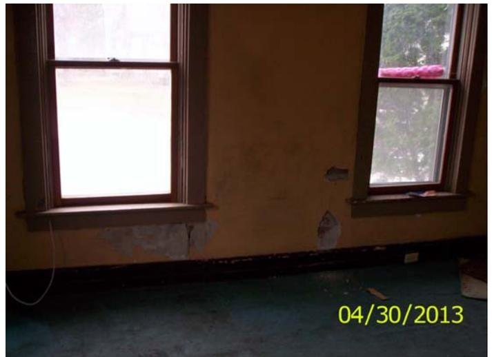
Water damaged walls
