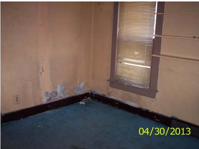
Water damaged wall
