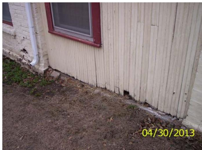
Rot damaged siding
