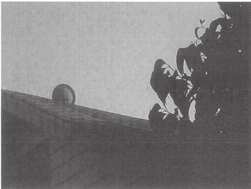
House Roof Northeast
