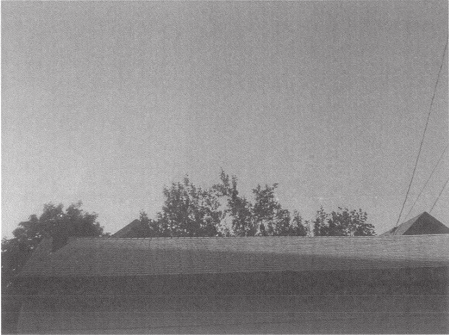
Garage Roof South
