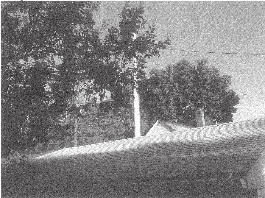
Garage Roof North
