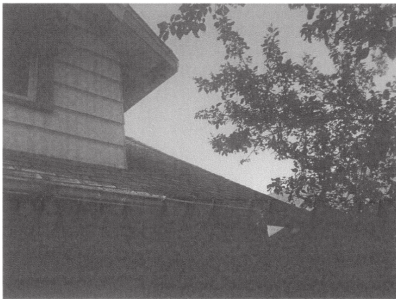
House Roof Southeast
