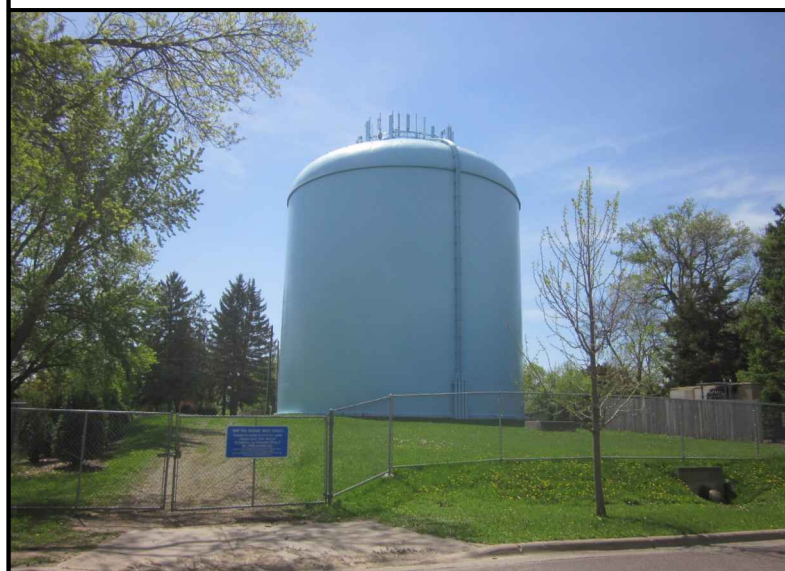
3 SITE OVERVIEW [LOOKING EAST]
