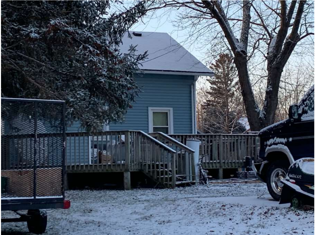
1071 Englewood Ave. Photos from recheck inspection on 12/2/24
