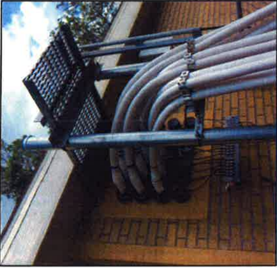
3 SHELTER COAX ENTRY SCALE: NONE
