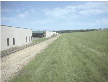
Back side of Levee near Holman Field.
