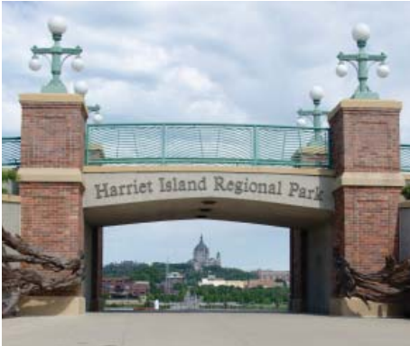
Harriet Island Regional Park Levee Entrance
