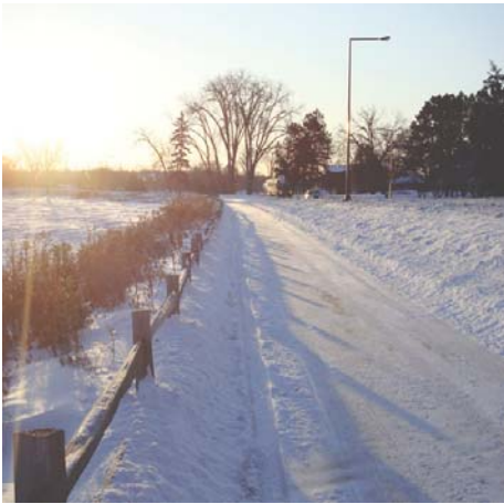
Trail maintenance will include snow plowing.
