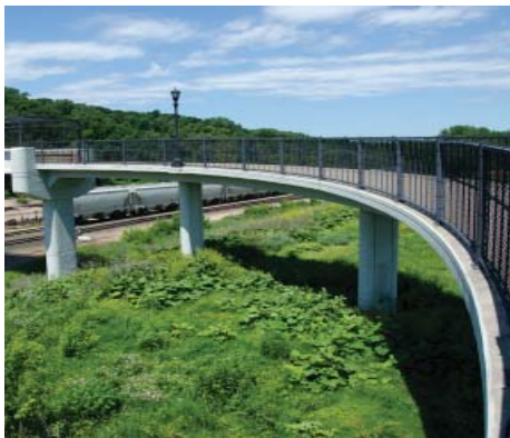
Bike & Ped Bridge in South St Paul connects to Dakota Co. Trail Systems.
