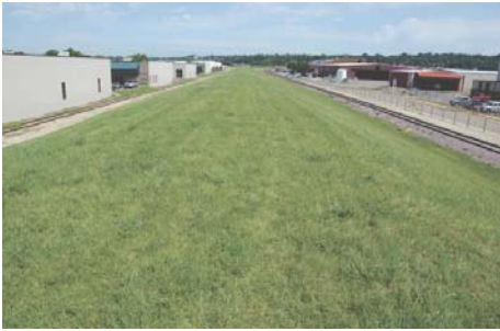
Top of levee along Airport Rd.
