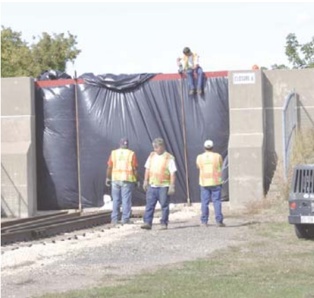
Preparing levee closure for flood conditions
