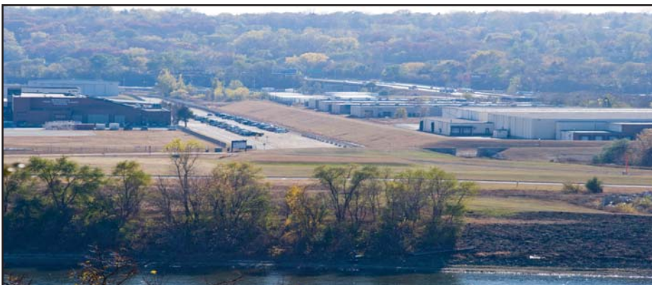
Levee view from Indain Mounds Park
