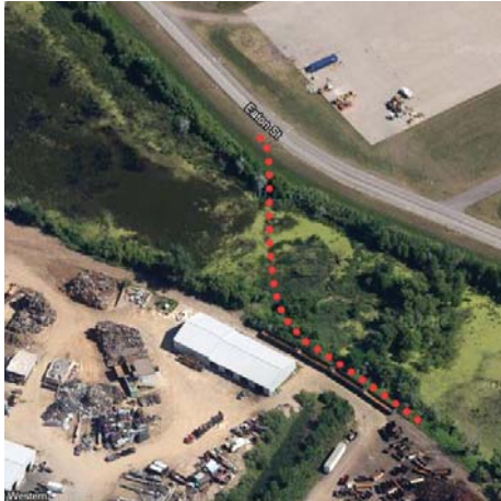
Wetland crossing Boardwalk location
