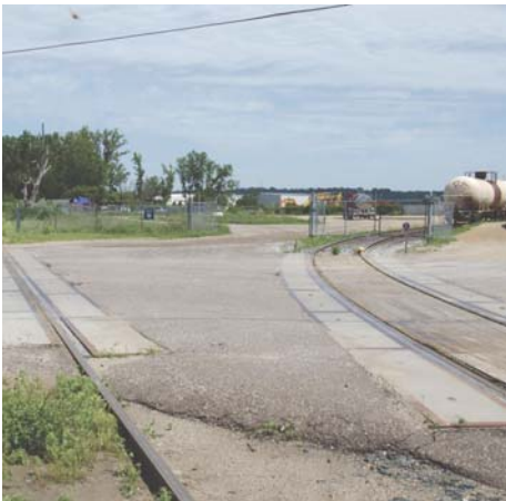
Track Crossings at Barge Channel Rd.
