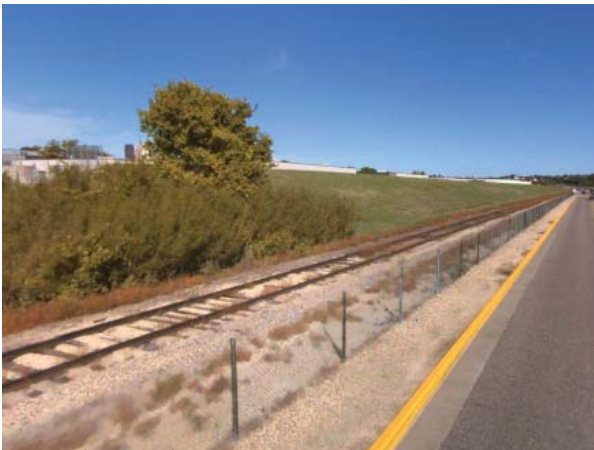
View of Levee from Airport Road
