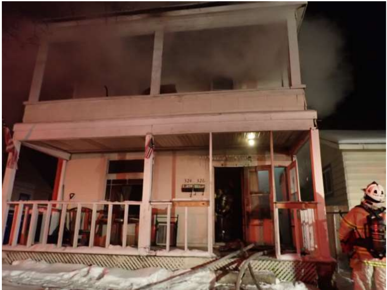
326 Charles Ave – Fire photos sent on 7/11/23
