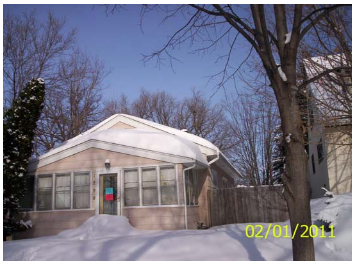
South and east sides, posting
