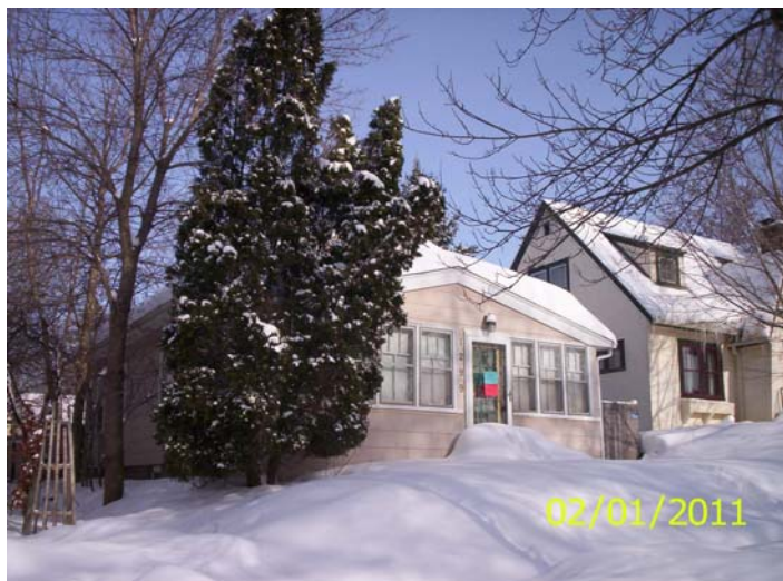
West and south sides, posting
