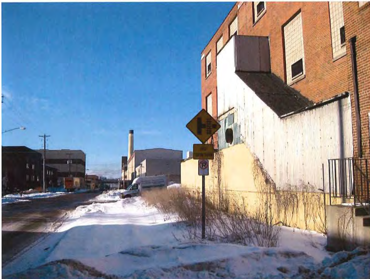
Looking west along Wabash, subject site on the right
