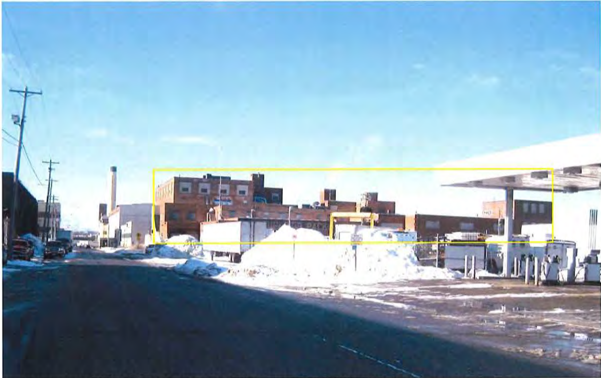
Looking west/northwest along Wabash, subject site is the brick building in yellow outline
