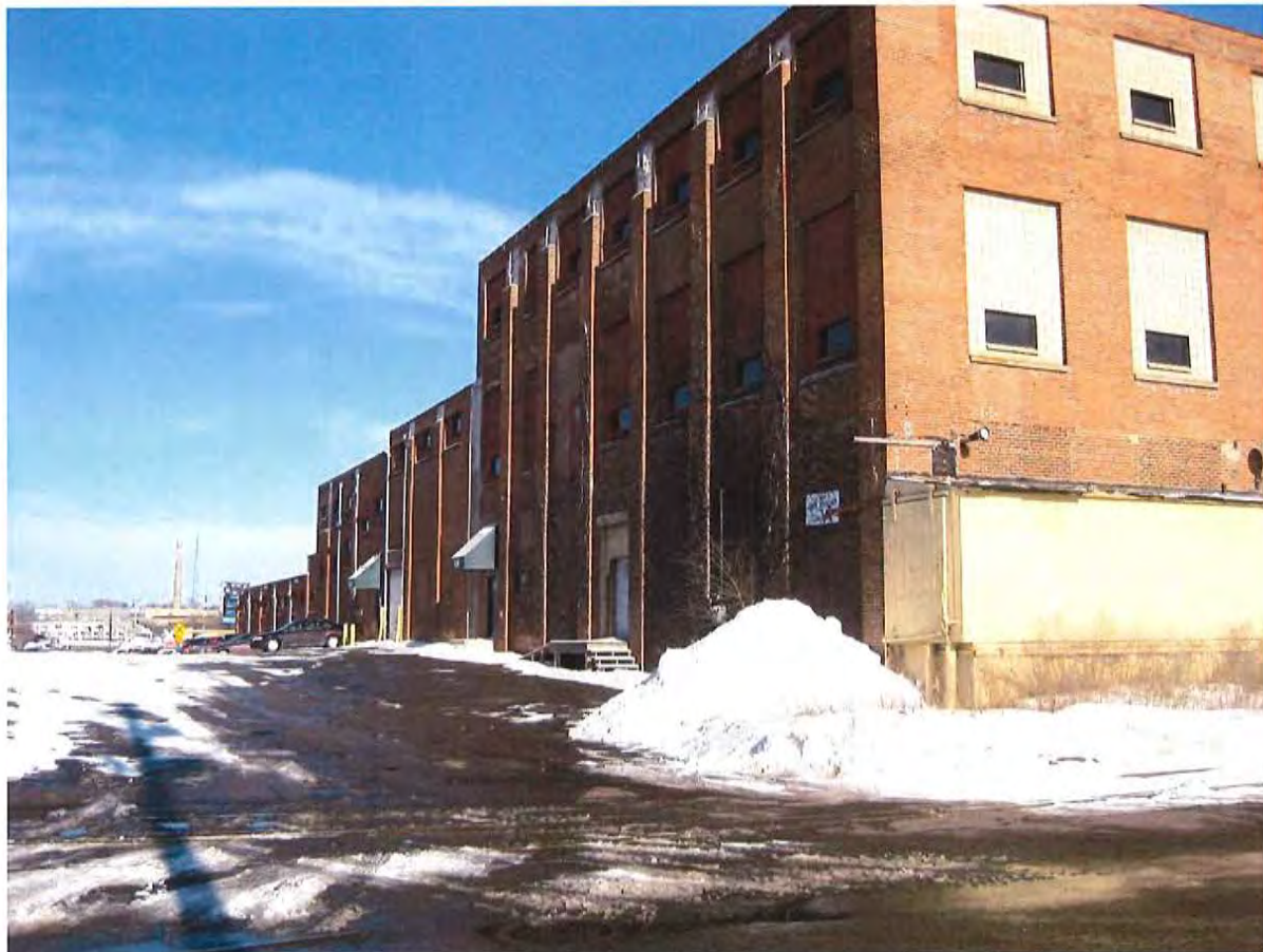
Looking north/northeast along Montgomery, subject site is the entire building and parking on right
