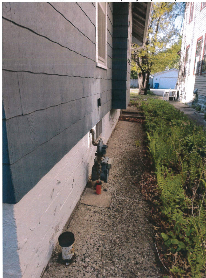
Photo #8 – Side of Building (May 13, 2021)
