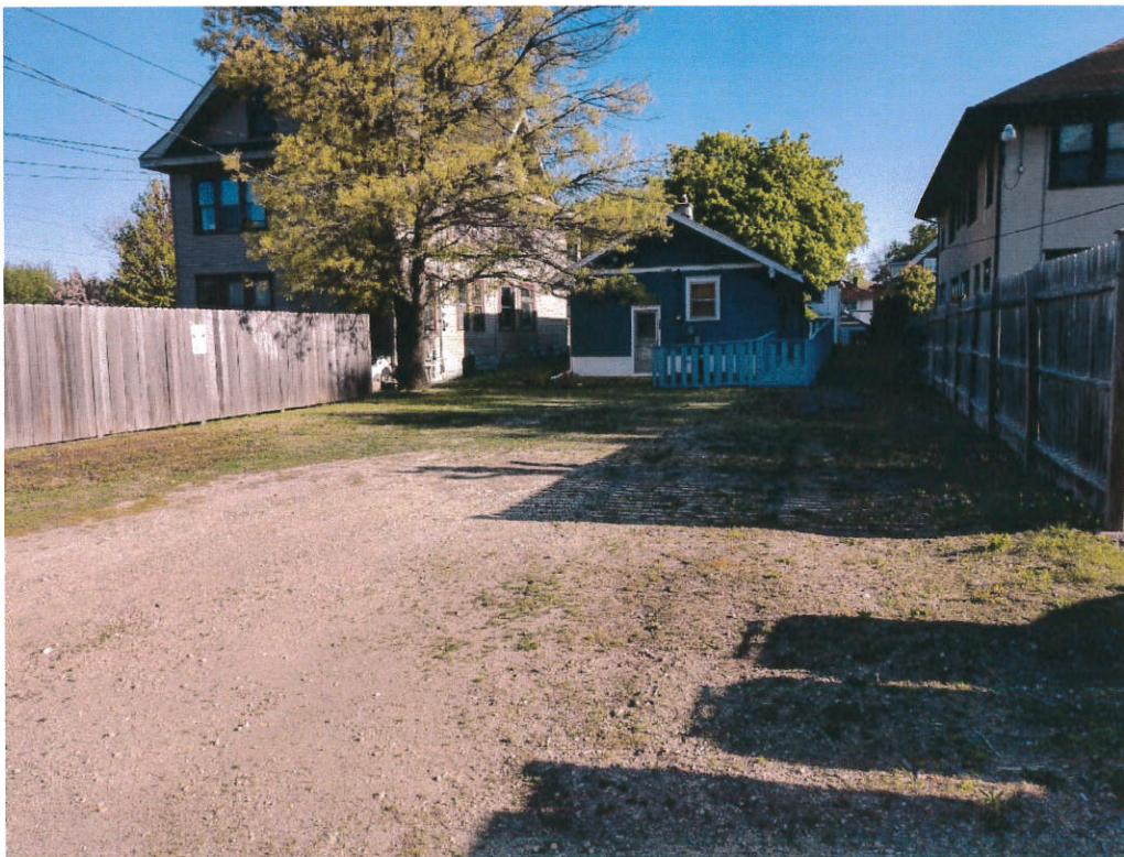
Photo #4 – Rear of Building (May 13, 2021)
