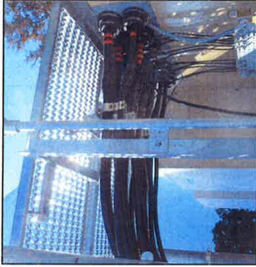
1 CABLE BRIDGE PHOTO SCALE: NONE
