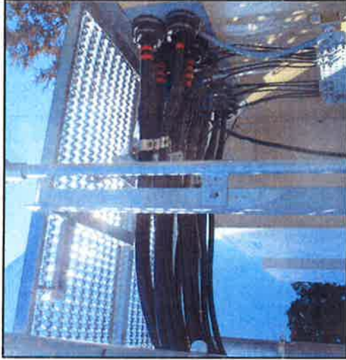
1 CABLE BRIDGE PHOTO SCALE: NONE
