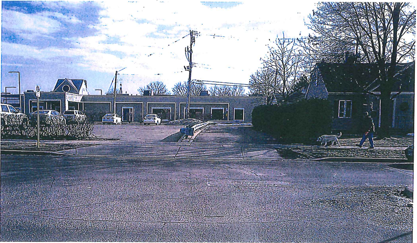
Looking south at site from across Highland: site, alley and adjacent single-family house.
