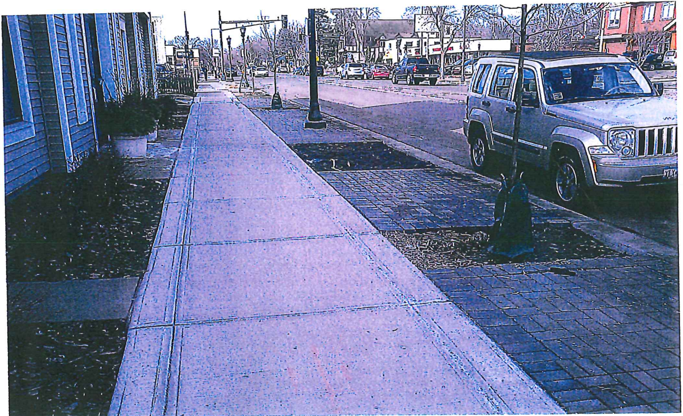
Street view of 2014 Highland sidewalk improvements
