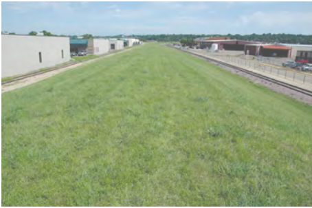
Top of levee along Airport Rd.
