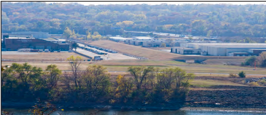
Levee view from Indain Mounds Park
