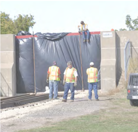
Preparing levee closure for flood conditions
