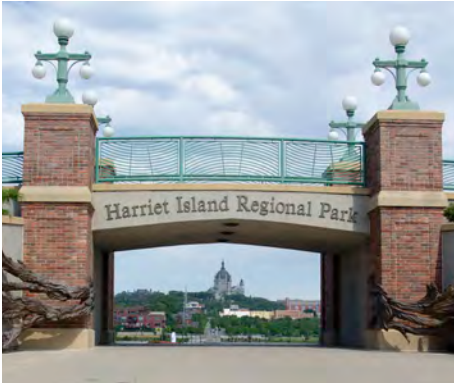
Harriet Island Regional Park Levee Entrance
