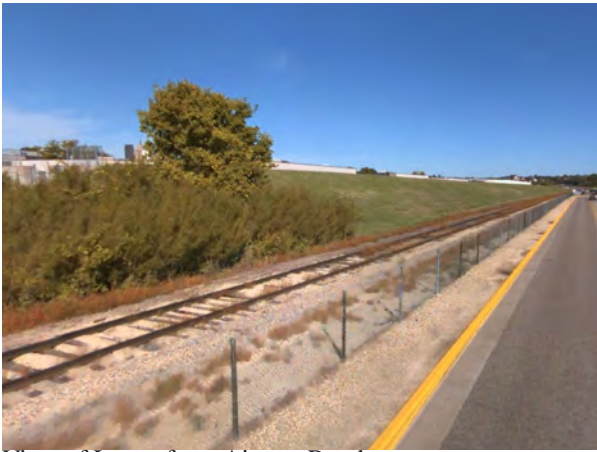
View of Levee from Airport Road
