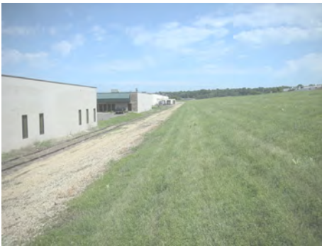
Back side of Levee near Holman Field.
