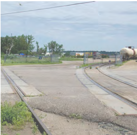
Track Crossings at Barge Channel Rd.
