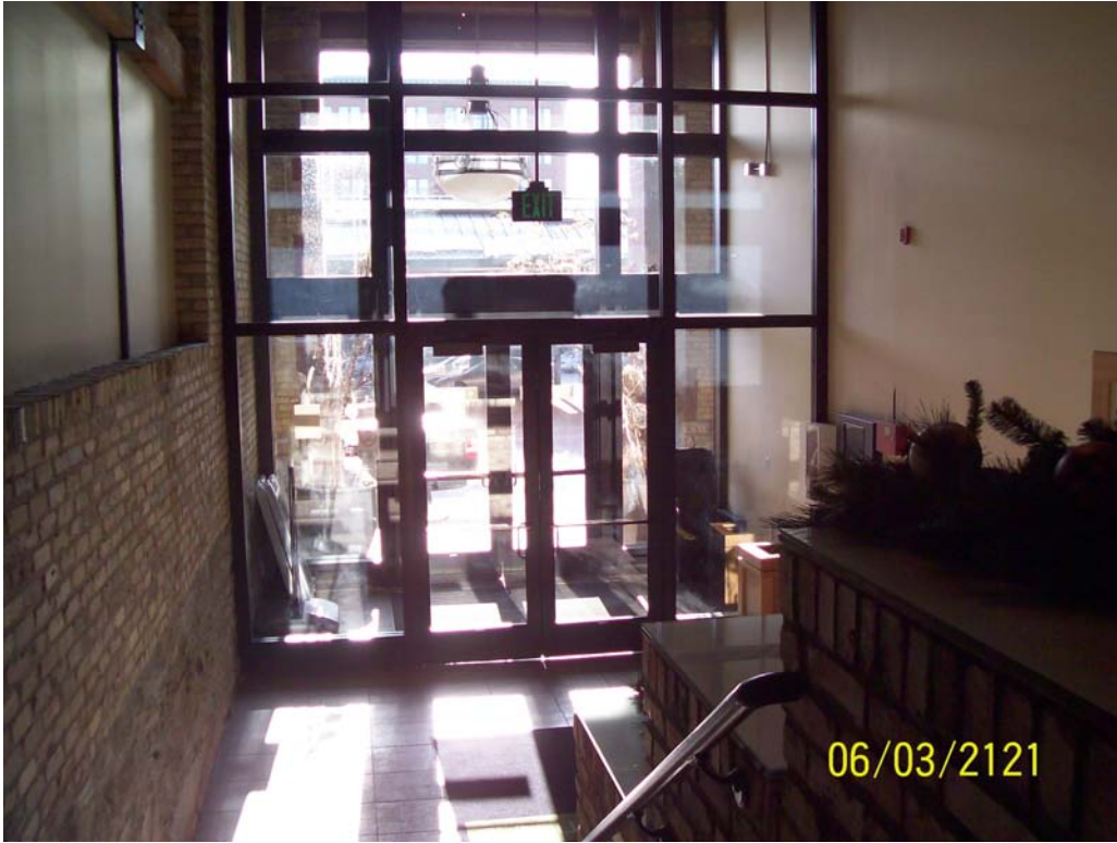
Front door. Pictures above are of the egress doors in questions and the front door.
