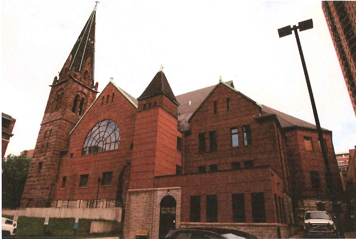
Figure 6 View from South side showing bell tower at left and hipped roof at right 7/27/15
