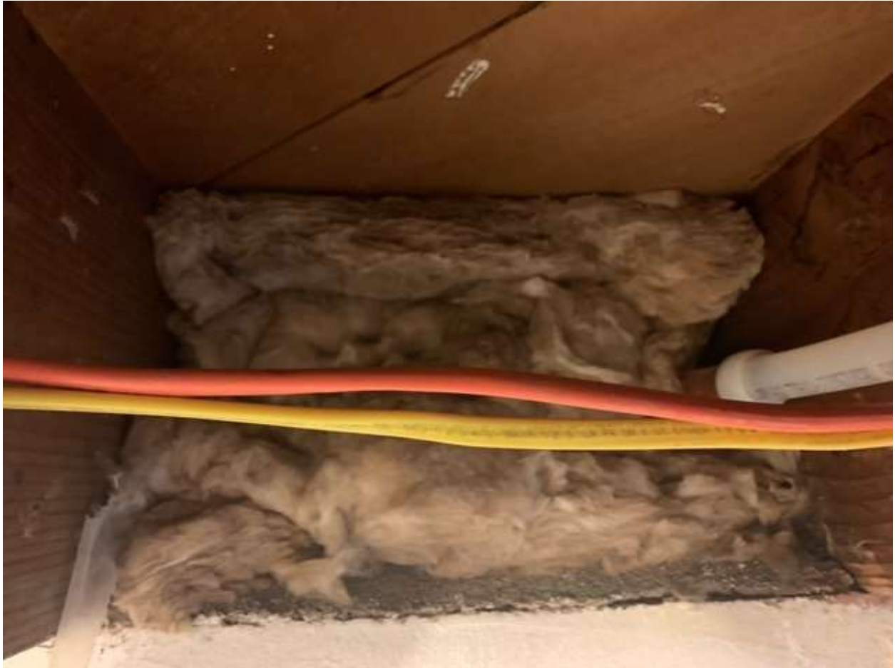
1457 Third St E.Chimney Sealed (Photos of old vents blocked off)
