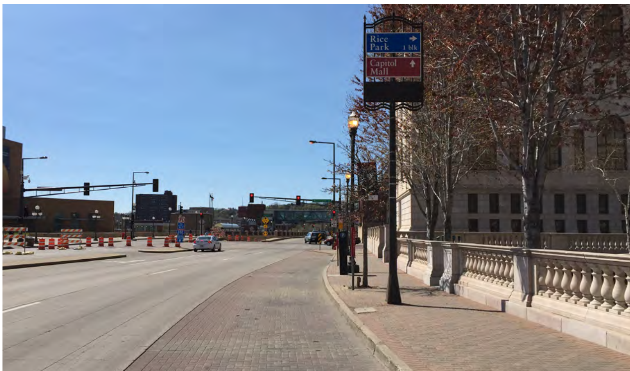
Existing conditions on Kellogg Boulevard.
