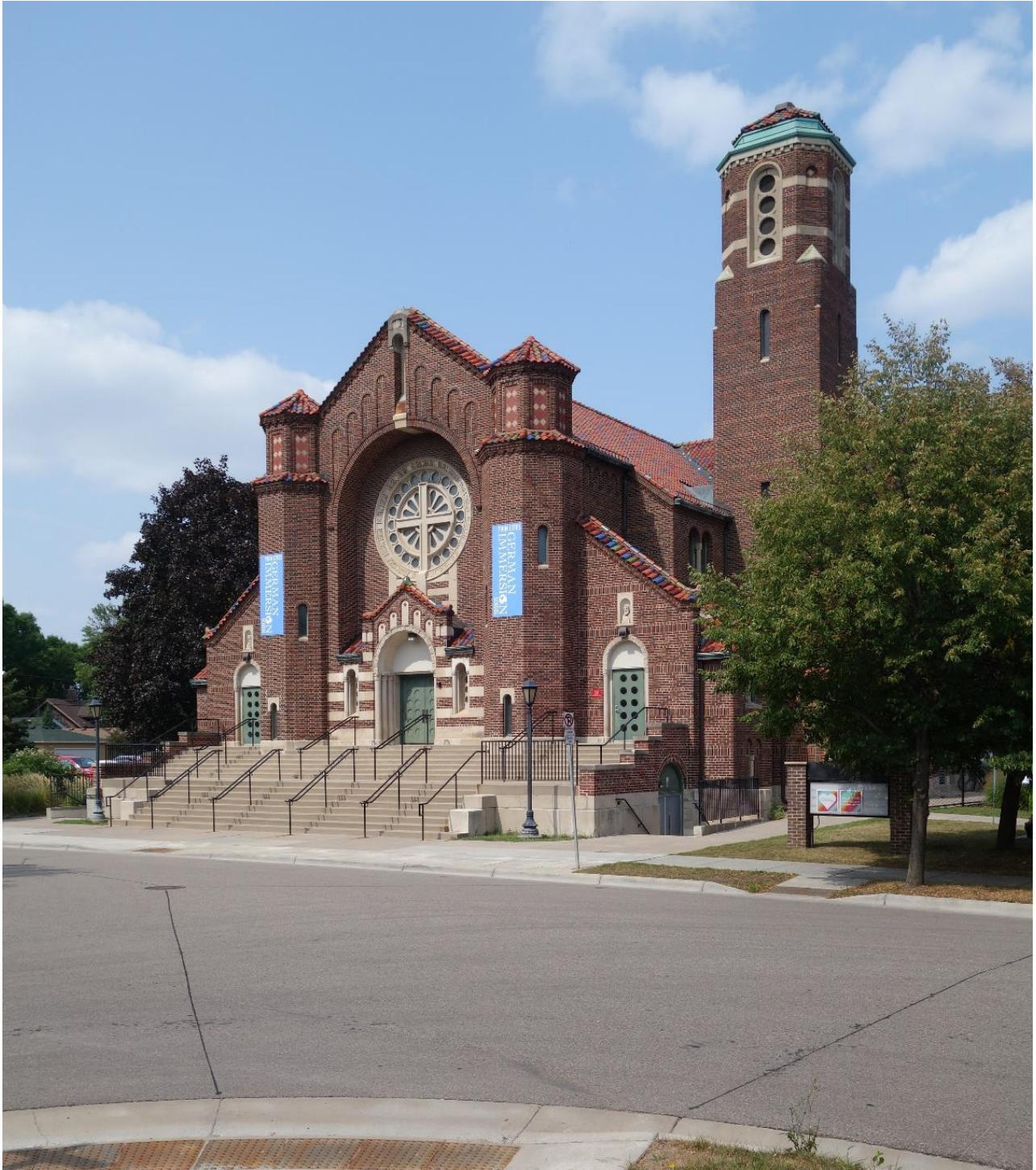
Figure 2. South elevation. Photo Rolf Anderson
