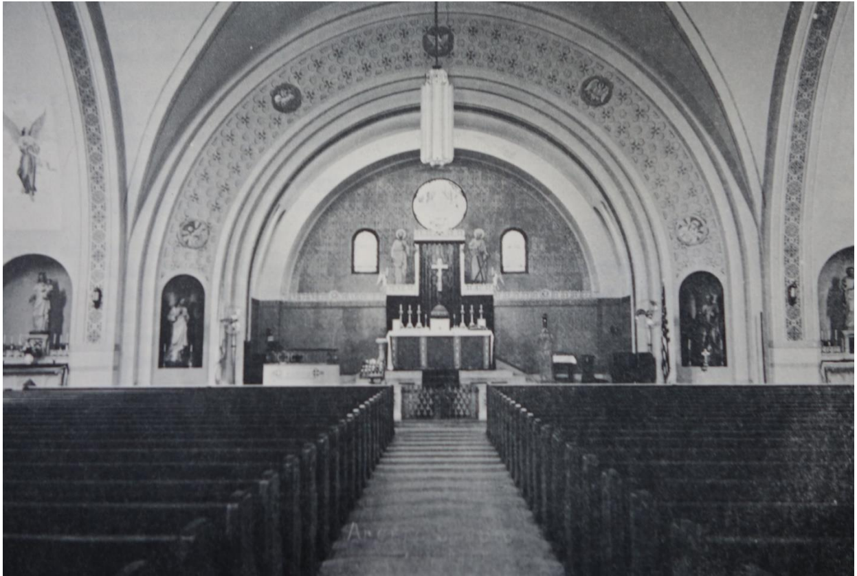
Figure 14. Historic interior view ca. 1930. Image St. Andrew's Archives
