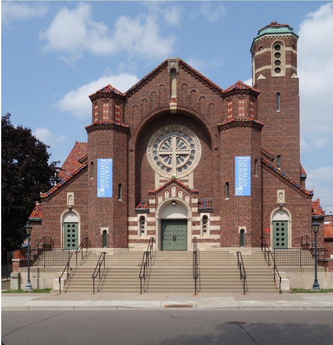
Figure 3. South elevation. Photo Rolf Anderson
