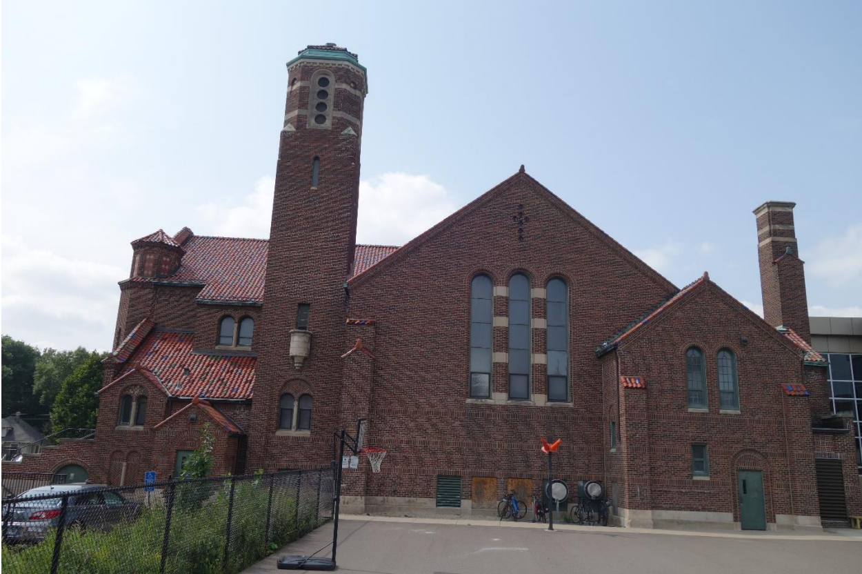
Figure 5. East Elevation. Photo Rolf Anderson
