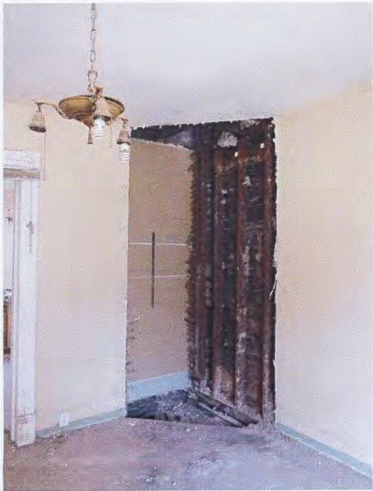
chimney demo 1 st floor
