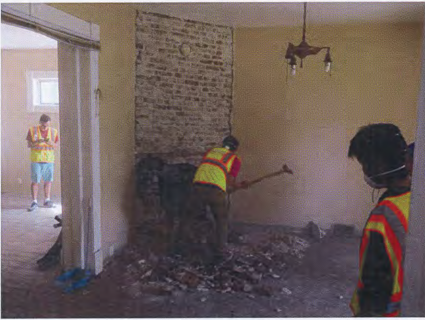
chimney demo 1 st floor
