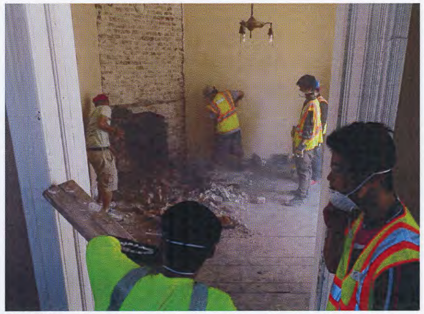
chimney demo 1 st floor
