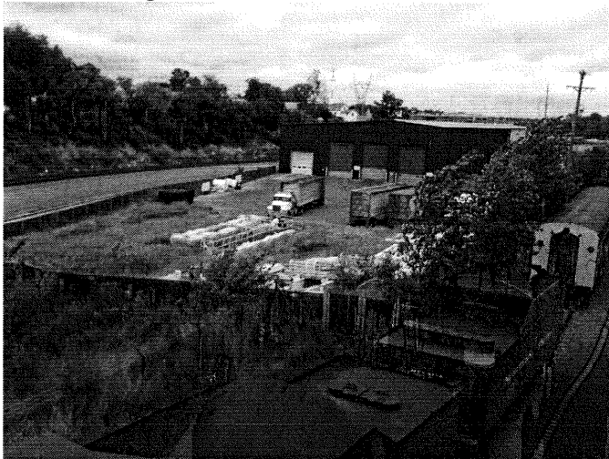
Second floor view of Waste Management west yard
