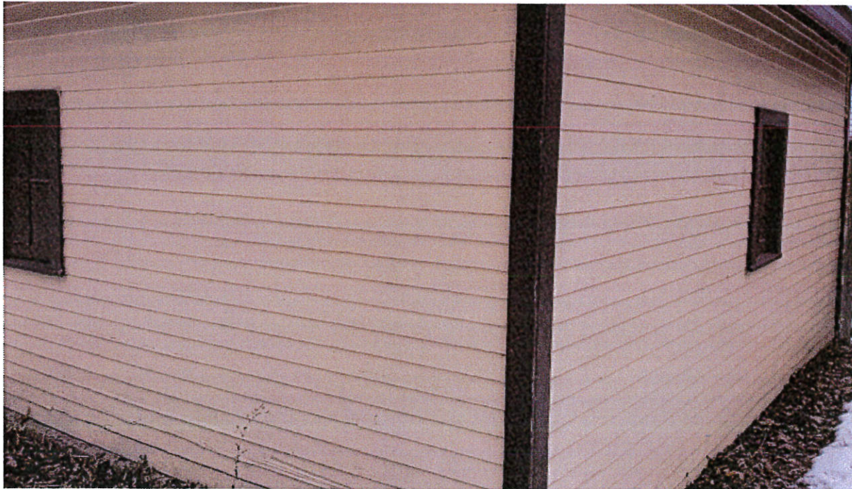
Image - picture of two walls of the garage:
