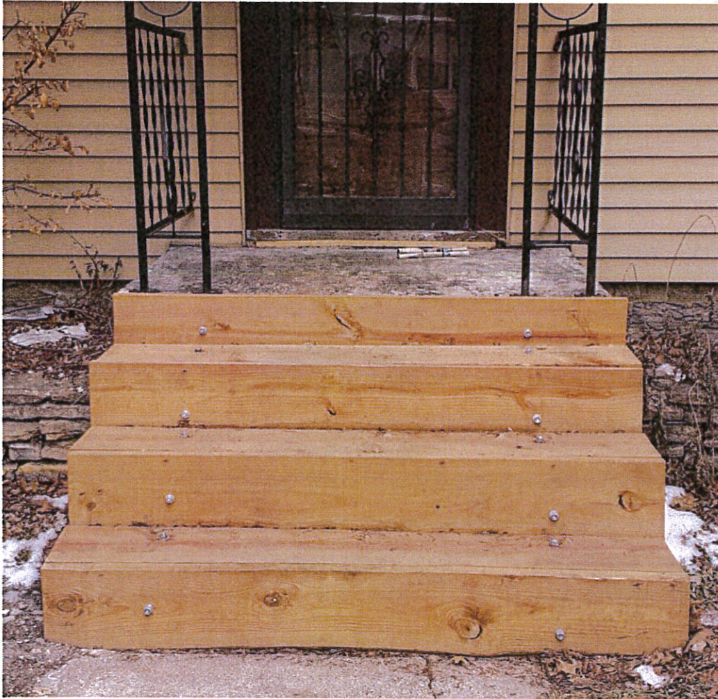
Image - wood-sheathed steps:
