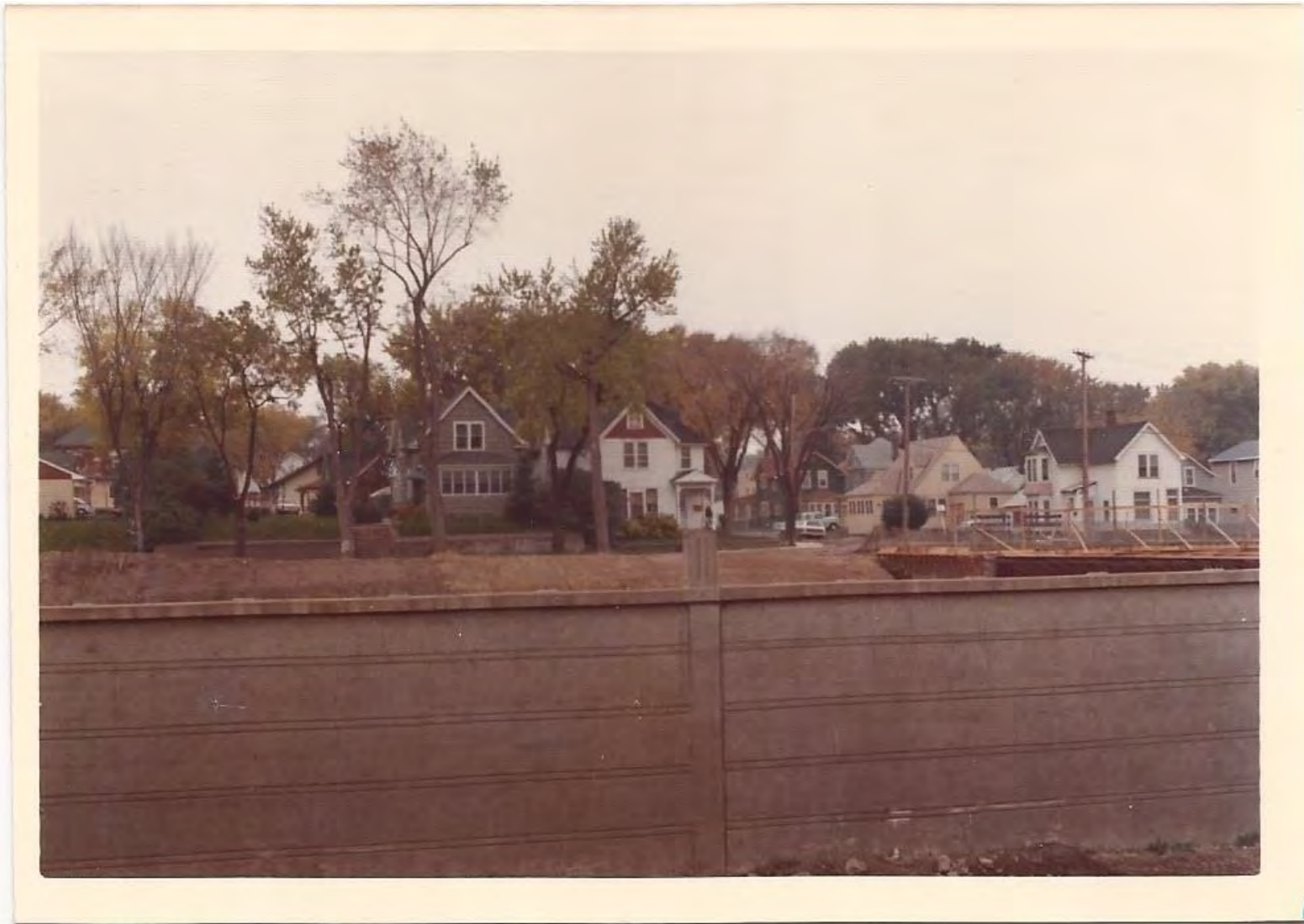
Circa 1973 photo showing retaining wall on downhill property
