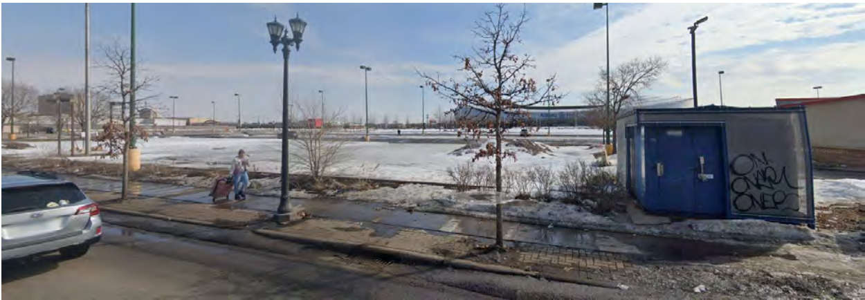
Project site includes portion of McDonald’s building and drive through lanes to the west, utility boxes too
