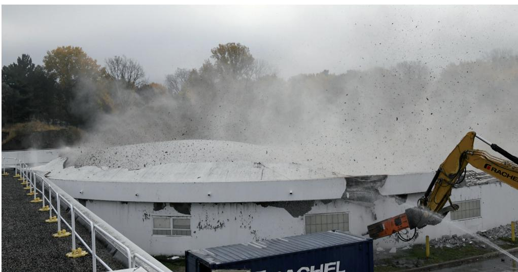
The historic dome on clarifier No. 2 came down on Thursday, October 30 after about an hour of demo work. Built in 1938, the dome was one of two that were added to the treatment plant to allow the solids built up from the softening process and flocculation to settle out. The sludge would sink to the bottom to be sent over to the thickening building while the clear water went on to the recarbonation basin to be treated. The clarifier room was a highlight of treatment plant tours for many years.
