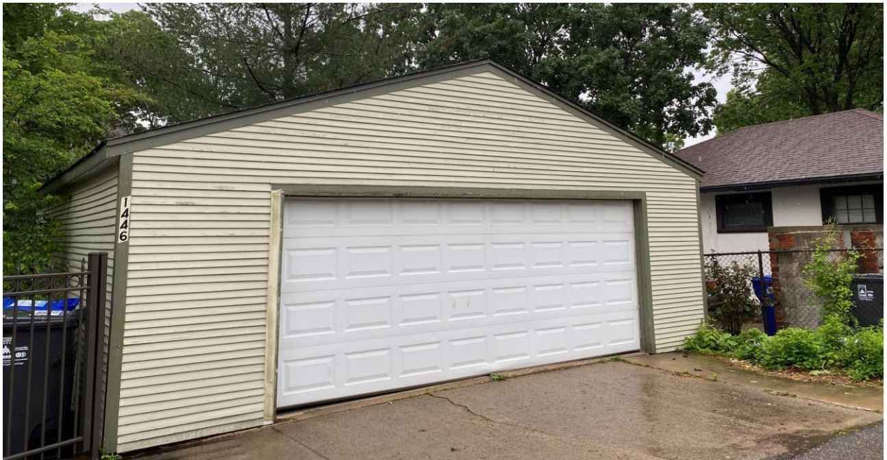
Garage that will be demolished
