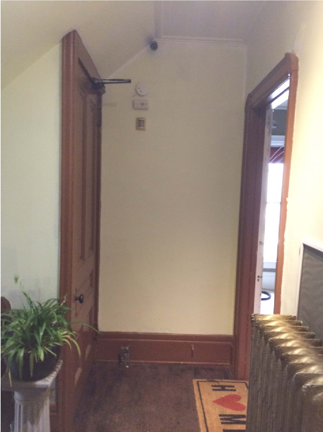
Hallway of 2 nd Floor
