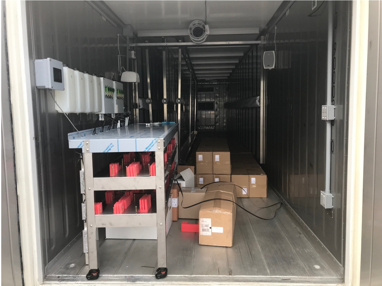
Figure A2: Interior photo of the MN Acre Farms hydroponic container farm on the morning of placement (August 28, 2020). The growing racks are apparent in the rear. The boxes contain the structures for the planting rows and hydroponic circulation tubing. The nutrient delivery pumps and seedling table are at left. It is important to stress that the final assembly of the farming system requires electricity and so we have as yet been unable to take these steps.
